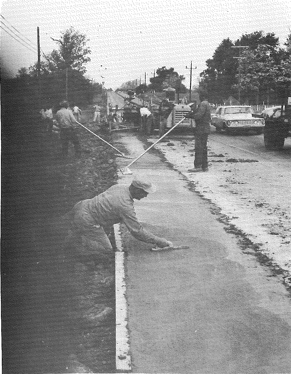
Figure 3. Finishing of Concrete on Widened Pavement on Lexington-Versailles Road.
