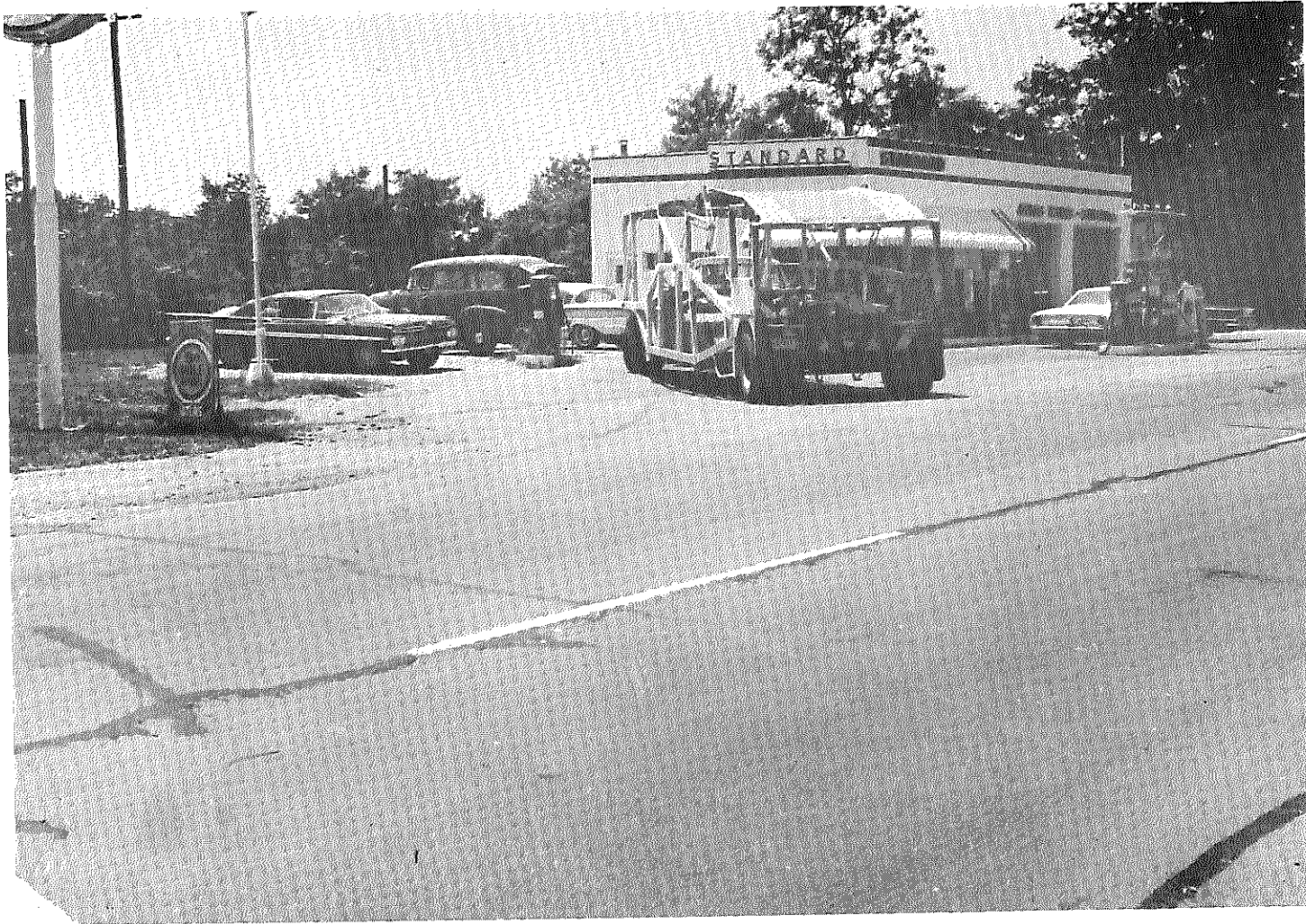
Figure 14. US 60, Shelbyville to Middletown, June 1964. A view of a section of the pavement nine months after sealing.
