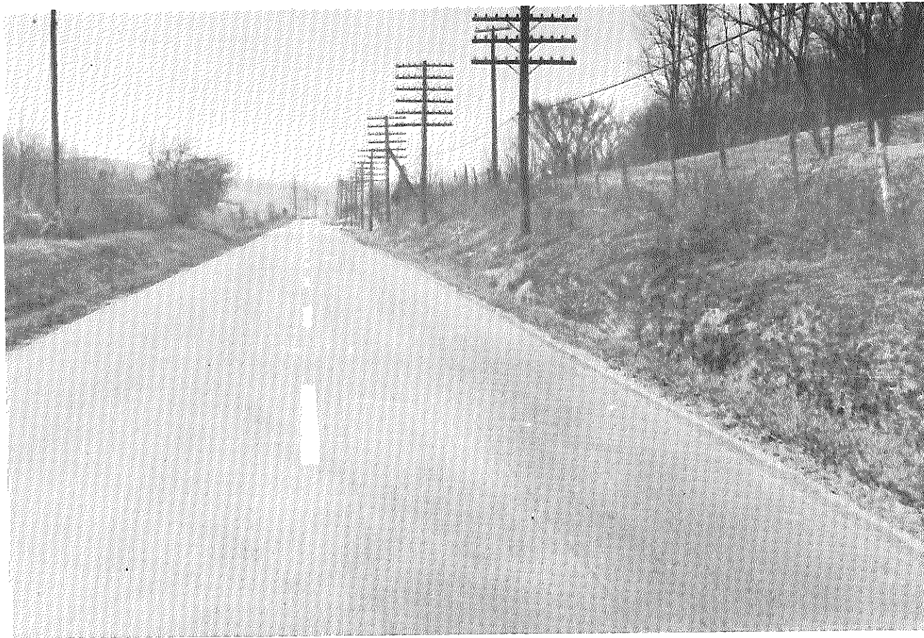
Figure 24. US 25, Georgetown to Williams- town, April 1965. This area had received a double application of slurry seal.
