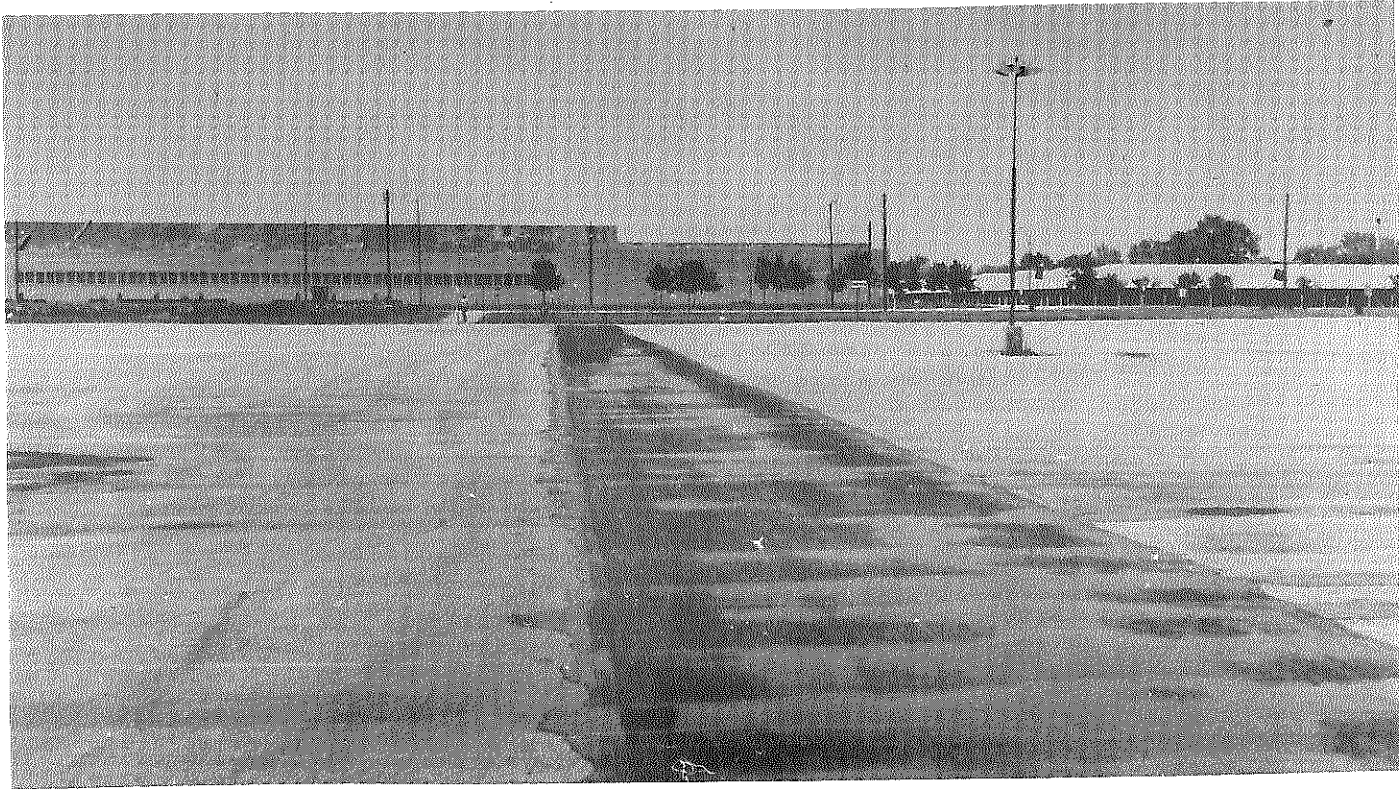
Figure 6. State Fair and Exposition Center, July 1963. The slurry laid thicker in depressed areas as a result of the wavy condition of the surface. Note the hot-mix bituminous patches elsewhere on the surface.
