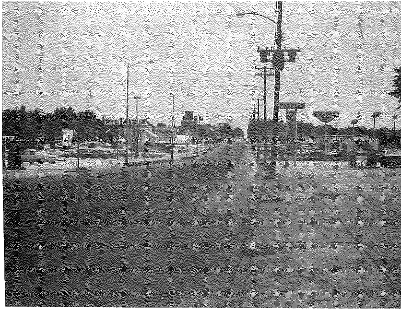
Figure 14. US 31-W, Bowling Green By-Pass. Tack coat was tracked onto the sand asphalt.
