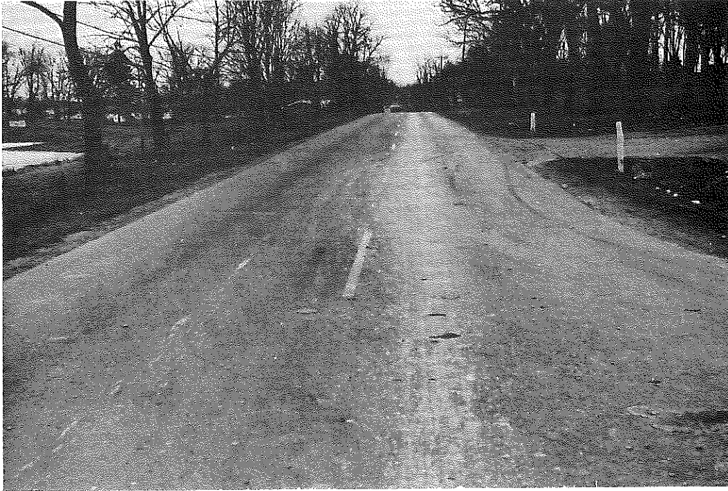
Figure 3. Lawrenceburg Fairgrounds Entrance on US 62 (looking east). Asphalt was tracked from the fairgrounds onto the sand-asphalt surface.
