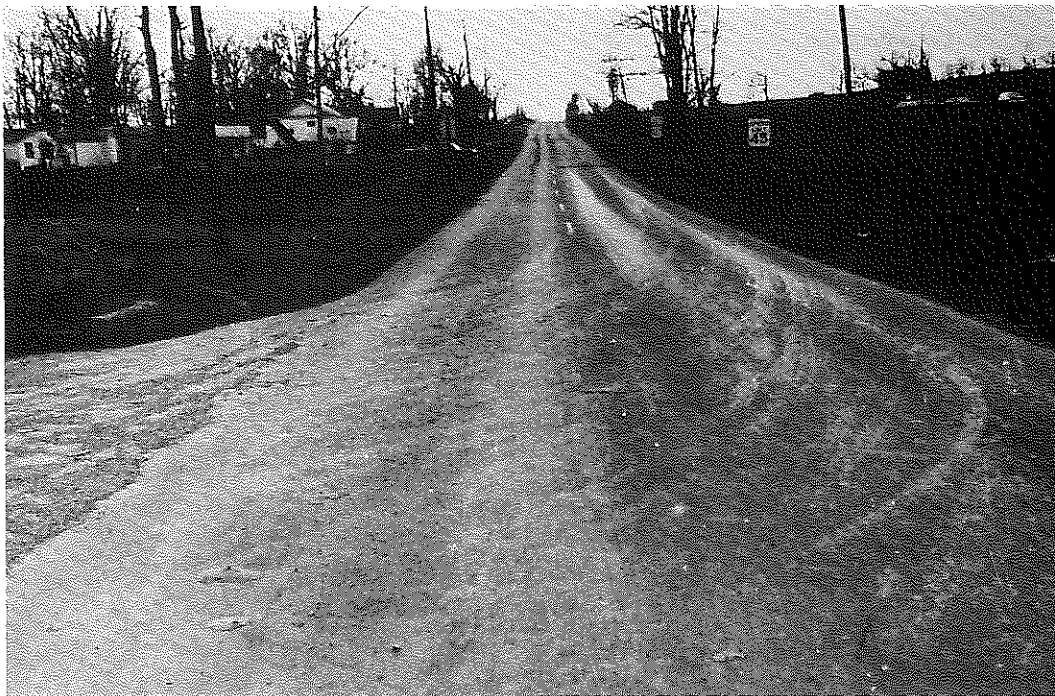
Figure 4. Lawrenceburg Fairgrounds Entrance on US 62 (looking west). Asphalt was tracked from the fairgrounds onto the sand-asphalt surface.
