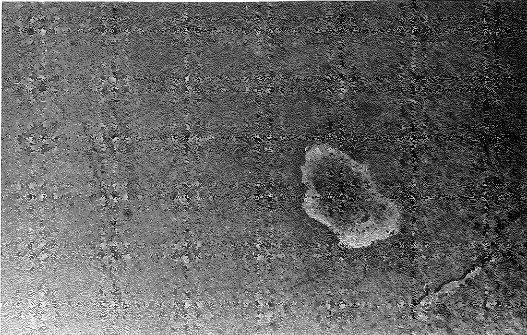
Figure 5. US 68, McCracken County. Note alligator cracks and sand-asphalt pop-out.
