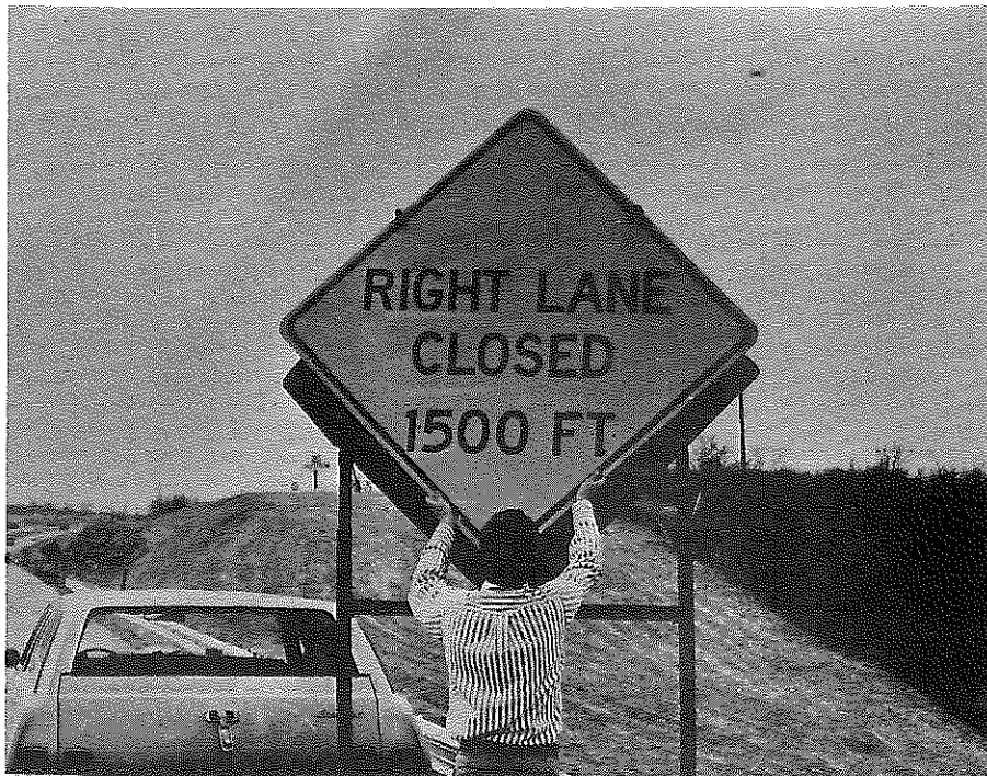
Figure 1. Research Personnel Positioning New Signs over Contractors' Signs.
