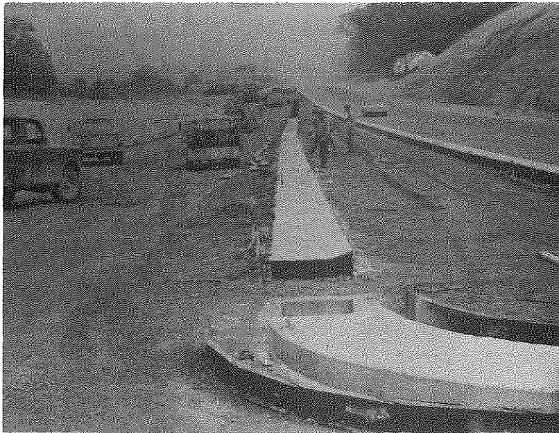
Figure 7. Construction of Lip Curve and Gutter Mountable Median
