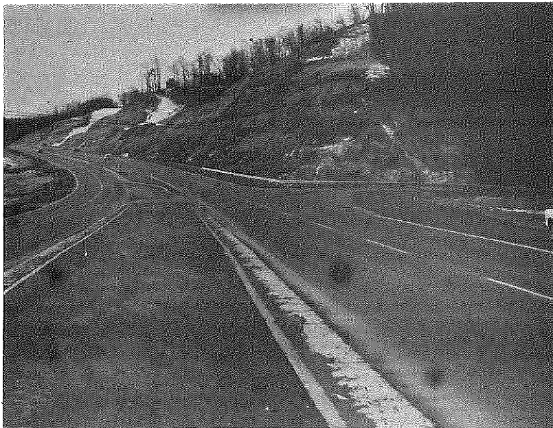
Figure 9. Lip Curve and Gutter Mountable Median
