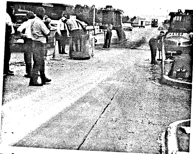
Figure 2. Handwork Used in Conjunction with the Cleaning Operation.
