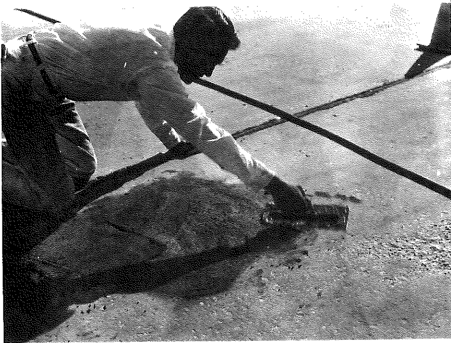
Figure 3. Patching the Deck
