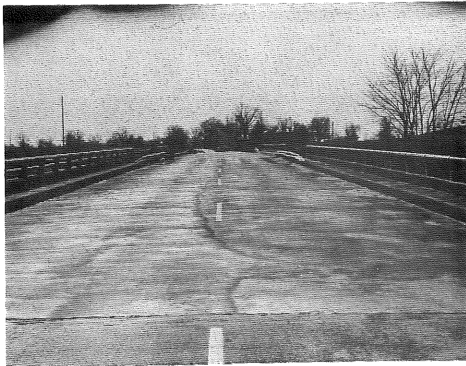
Figure 21. General Appearance of the Shelby County Bridge Deck, December 29, 1971
