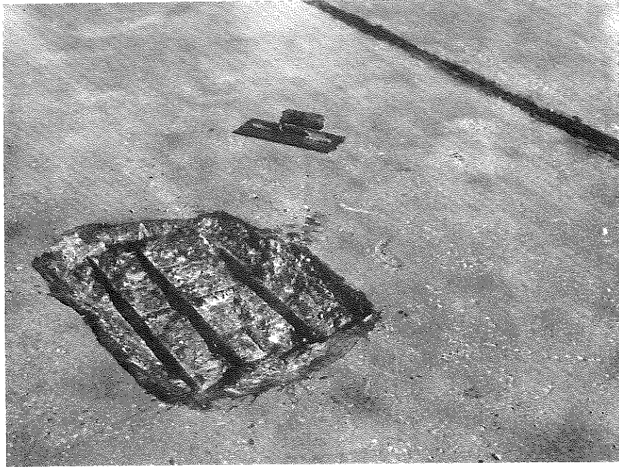
Figure 6. A Primed Patch Hole
