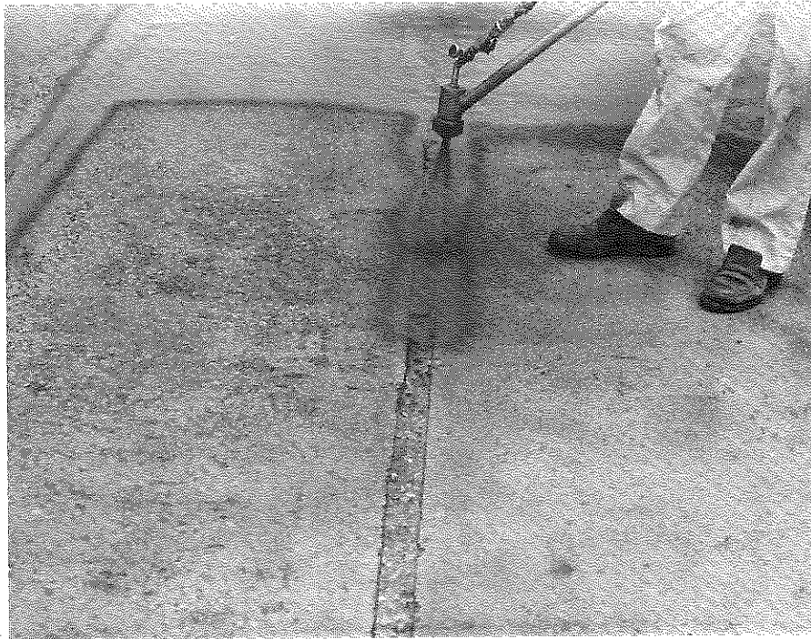
Figure 7. Spraying of the Clay City Deck
