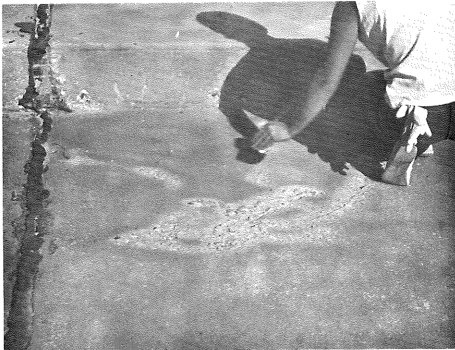
Figure 5. Priming the Patch Holes before Patching
