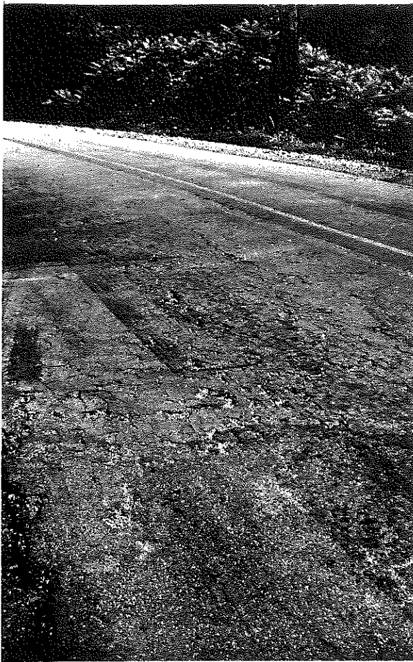
Figure 36. Section of US 60 between Olive Hill and Grayson; 1948 (14).
