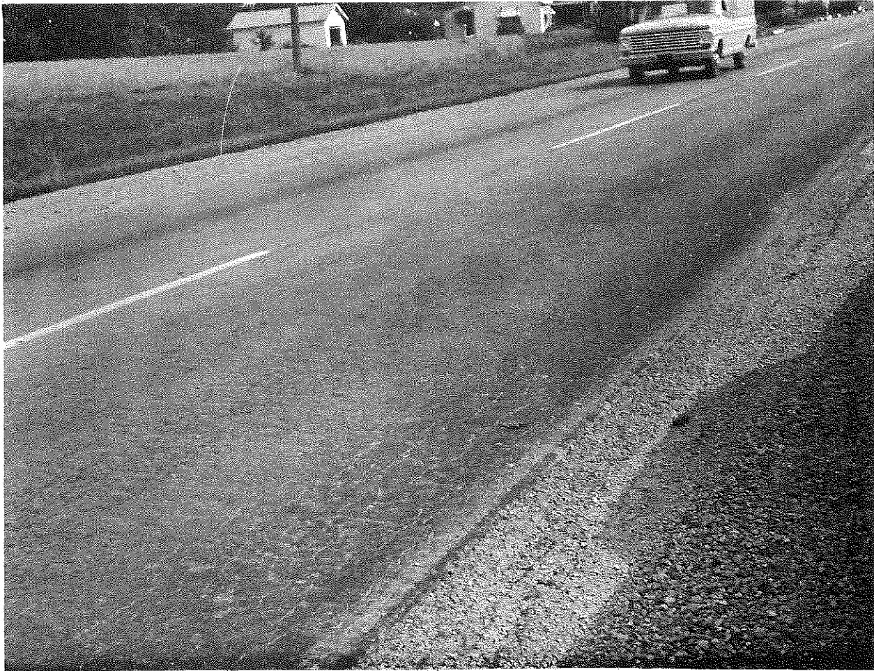
Figure 49. US 31 W North of Tennessee Line; Non-Reinforced, 8-inch Slab, No Joints; Built Experimentally in 1949; Carried Heavy Traffic until I 65 Opened; Source of Aggregate Unknown; June 6, 1968.
