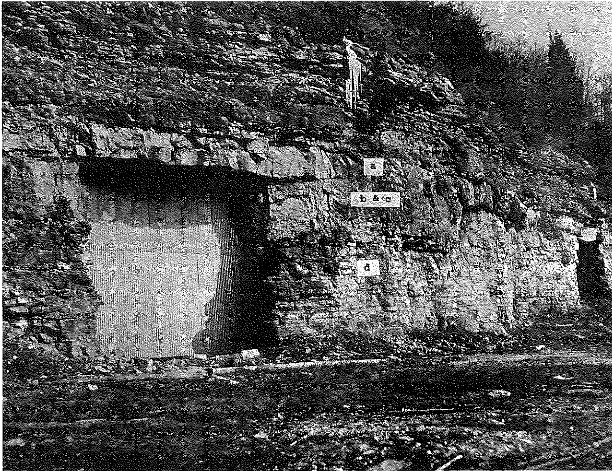
Figure 46. Old Tygart Limestone Company's Quarry and Mine at Lawton, Kentucky. Mine is now used to grow mushrooms. Proximity to Olive Hill quarry and poor performance of this aggregate on KY 32 invited investigation; February 10, 1972.
