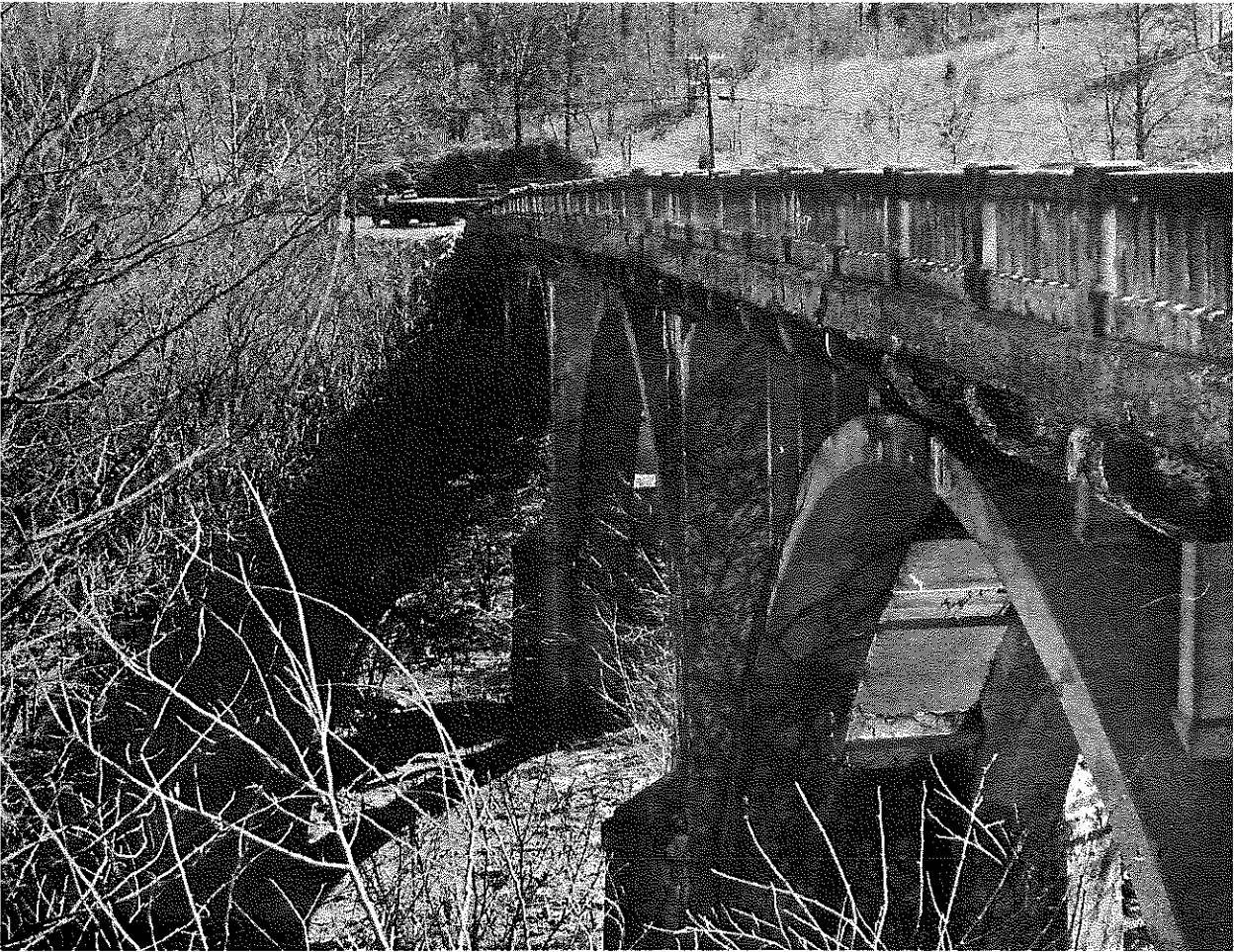
Figure 48. Tygart's Creek Bridge, US 60, East of Olive Hill; Built about 1927; March 1972.
