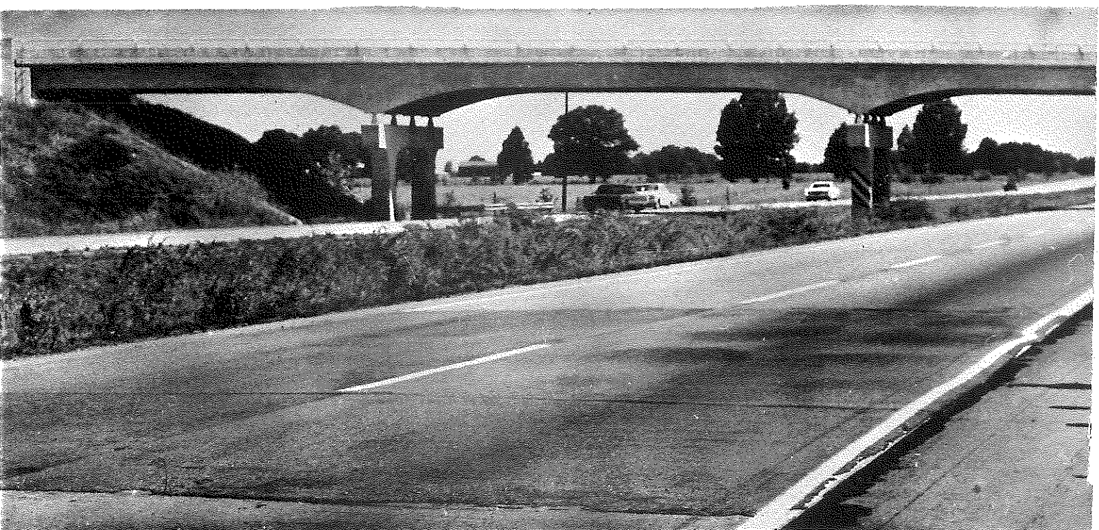
Figure 8. Same Site as above with Bituminous Patch, Station 280+75 NB; July 17, 1970.
