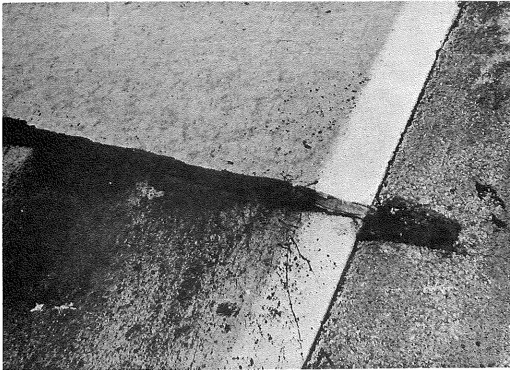
Figure 5. Closure of Relief Joint, Station 707+75 NB; July 15, 1968.
