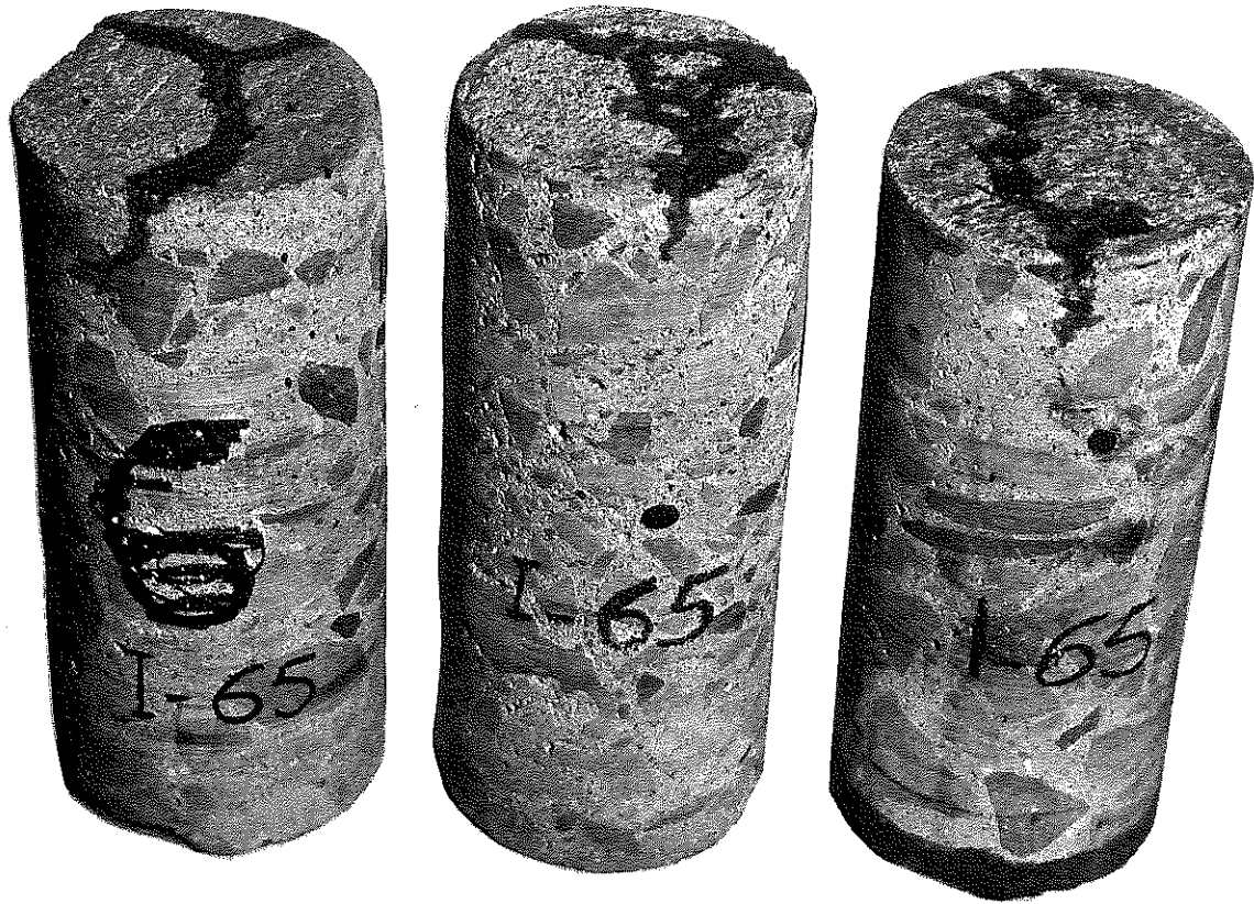
Figure 14. Cores Showing Cracks at Surface and Depth. Cracks have been wetted. Note indentation in surface of core at right; these appear to be finger imprints and suggest that someone recognized the crack before the concrete hardened. Note too that this crack is directly over a strand of steel (blackened).
