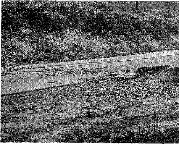
Figure 41. Blowup on KY 32; June 1950.
