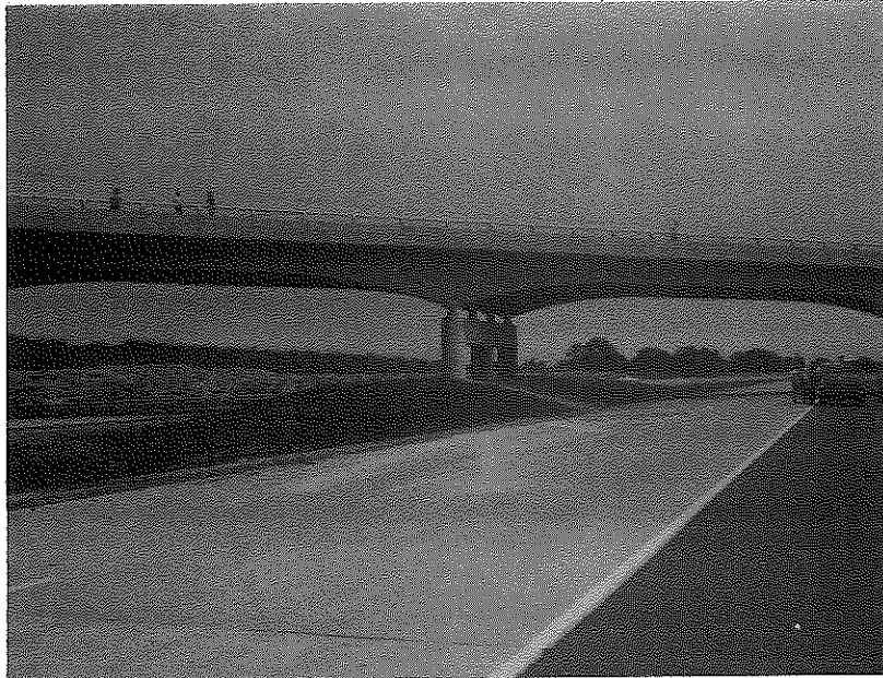
Figure 7. Median Bridge Piers "Protected" with Earth Berm.
