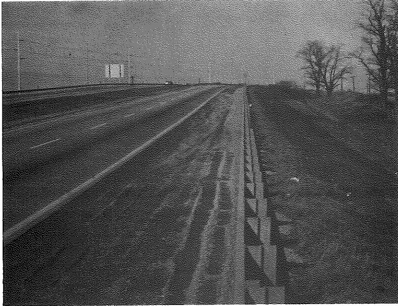
Figure 1. Steep Sideslope "Protected" with Guardrail.
