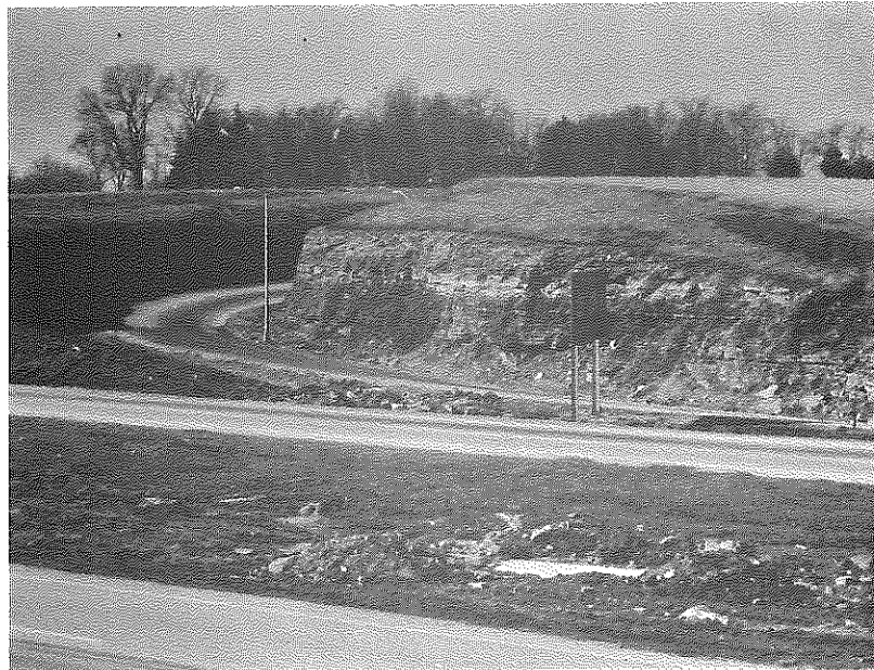
Figure 12. Elimination of Hazardous Gores by Contour Grading.
