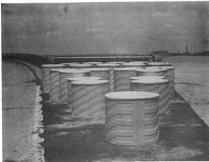
Figure 14. Fitch Type Impact Attenuator.
