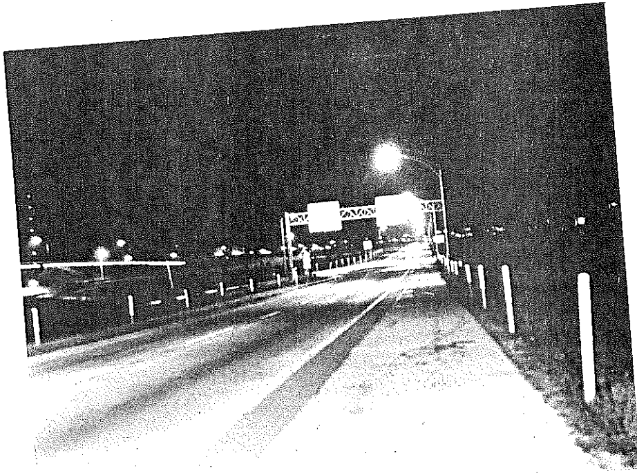
Figure 19. Typical Amber Delineator Placement
