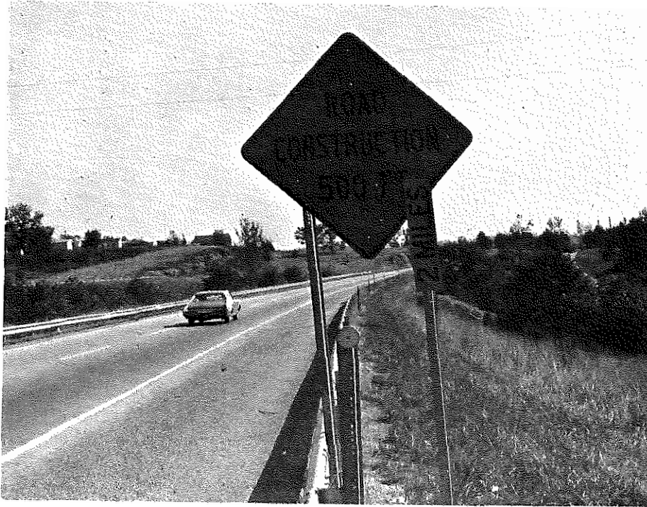
Figure 14. Errors which Cause Confusion and Disrespect for Warning Signs.
