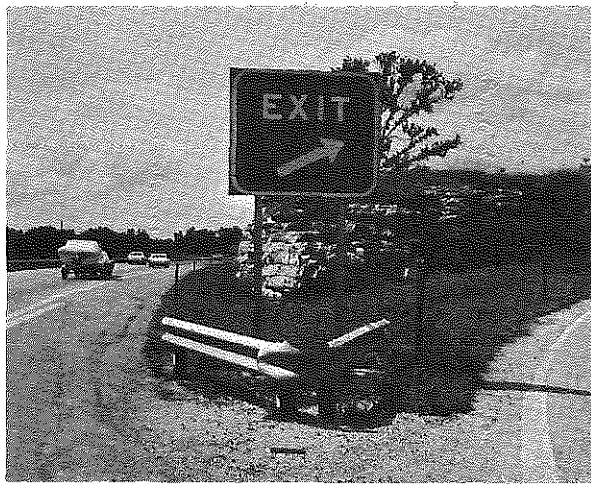
Figure 19. Location 10 before Contour Grading.
