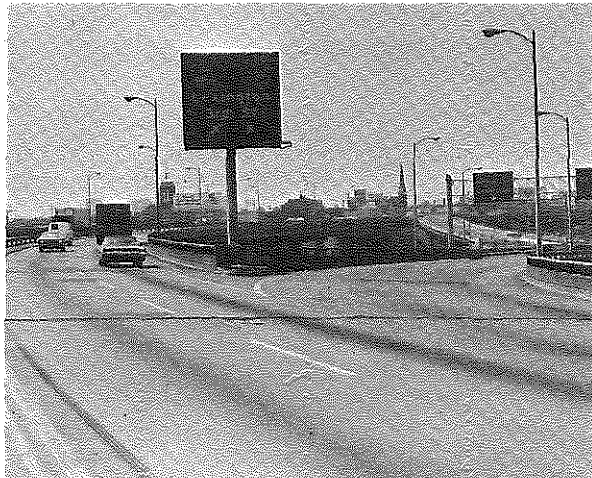
Figure 8. Location 3(d) before Installation of a HI-DRO Cushion.
