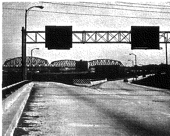
Figure 36. Location 3(b) Prior to Installation of the HI-DRO Cushion.
