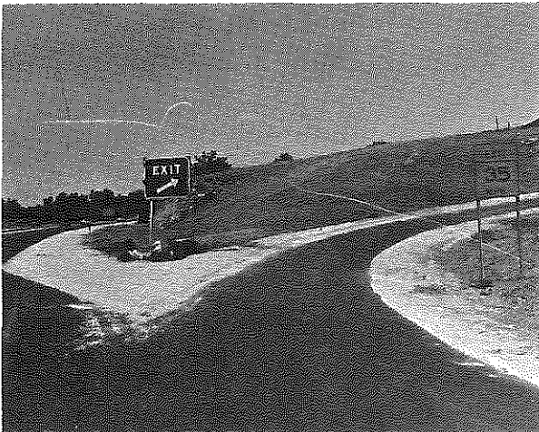
Figure 20. Location 10 after Contour Grading.
