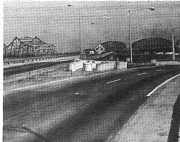
Figure 7. Fitch Inertial Barrier Installation at Location 3(c).
