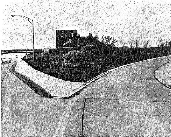
Figure 14. Location 8(a) before Contour Grading.
