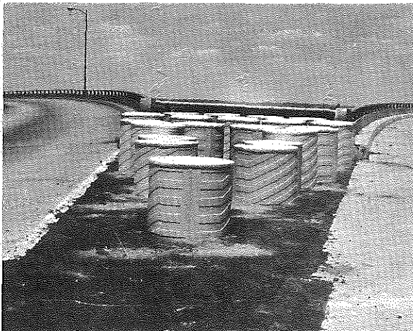
Figure 25. Fitch Inertial Barrier Installation at Location 14.
