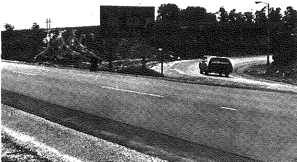
Figure 29. Location 18 after Contour Grading.
