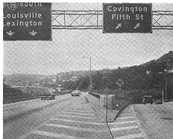
Figure 37. Location 7 Prior to Installation of the Fitch Inertial Barrier.
