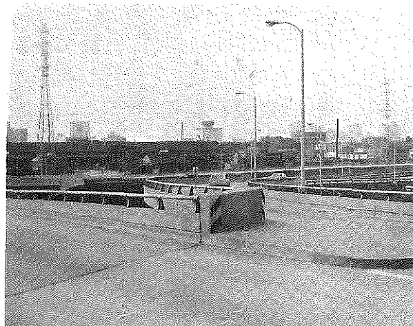
Figure 34. Location 3(a) Prior to Installation of a HI-DRO Cushion System.
