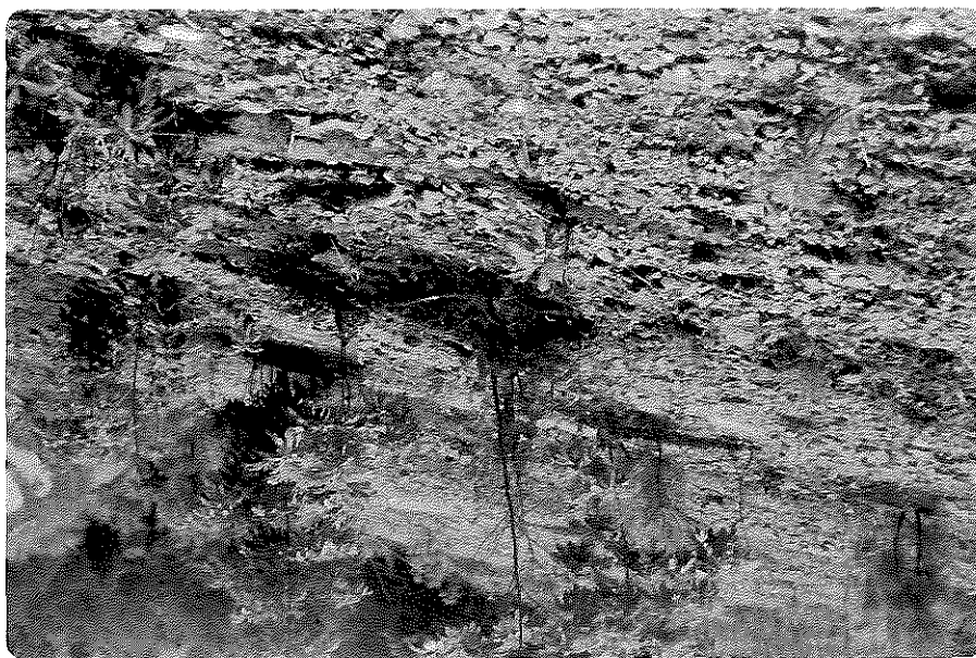
Figure 3-2/1. Pine seedlings growing on an eroded roadside slope 1 1/2 years after direct seeding.
