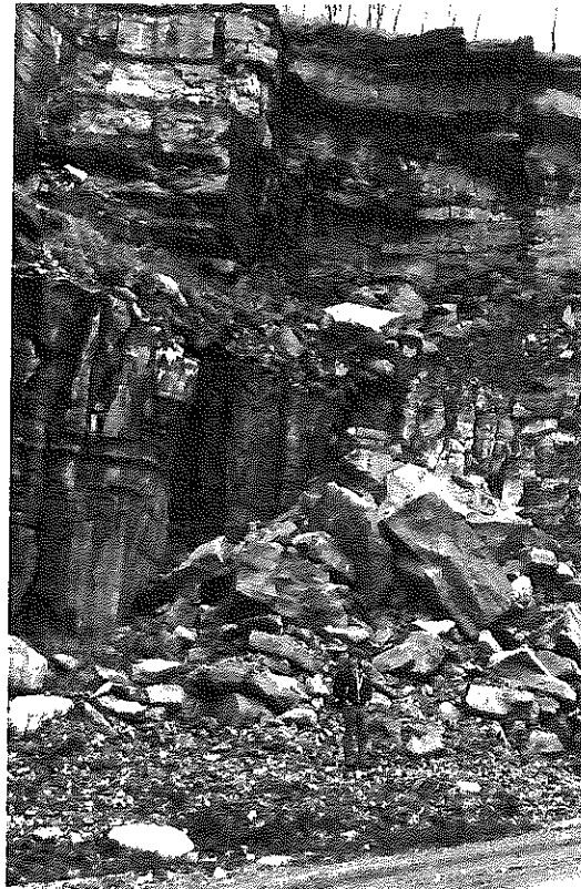
Figure 1. Poor Excavation Technique.
