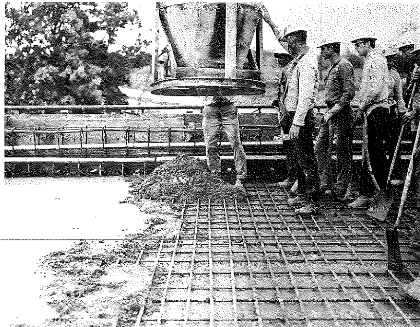
Figure 7. Placement of the Second Lift of the Bi-Layered Deck.
