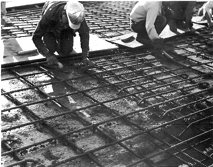
Figure 5. Finishing the First Layer of the Bi-Layered Deck.
