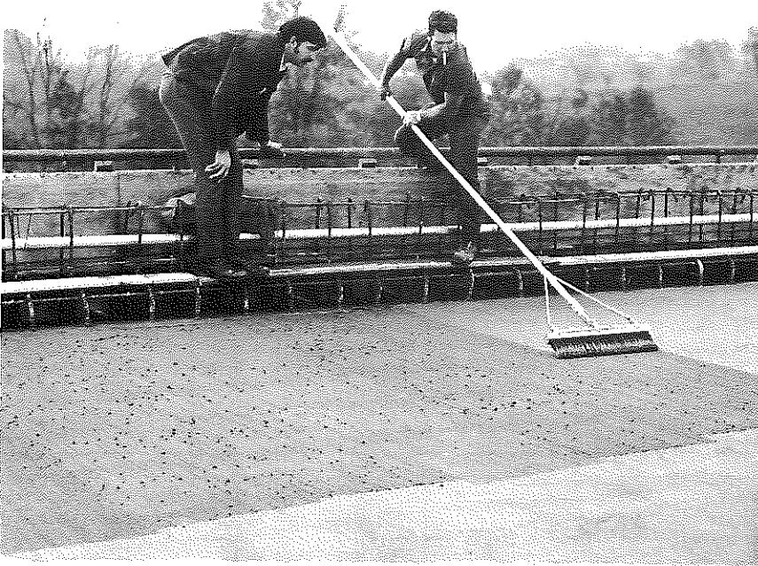
Figure 2. Transverse Brooming on the Eastbound, I-64 Bridge over US 60, Bi-Layered Deck.
