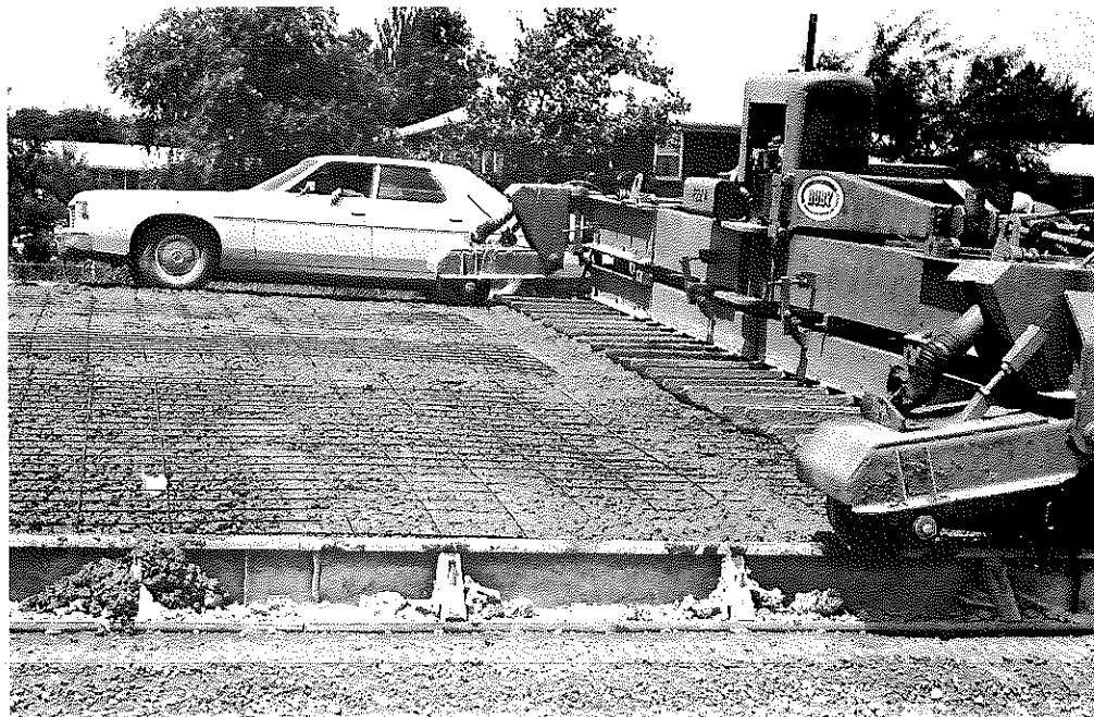
Figure A-2. Mainline Paving.
