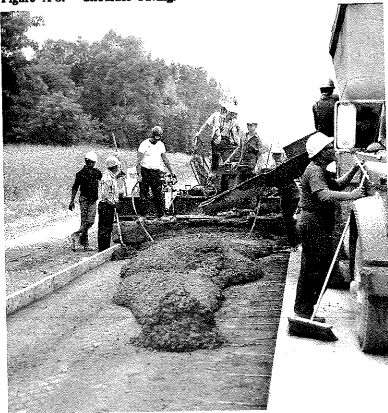
Figure A-8. Shoulder Paving.
