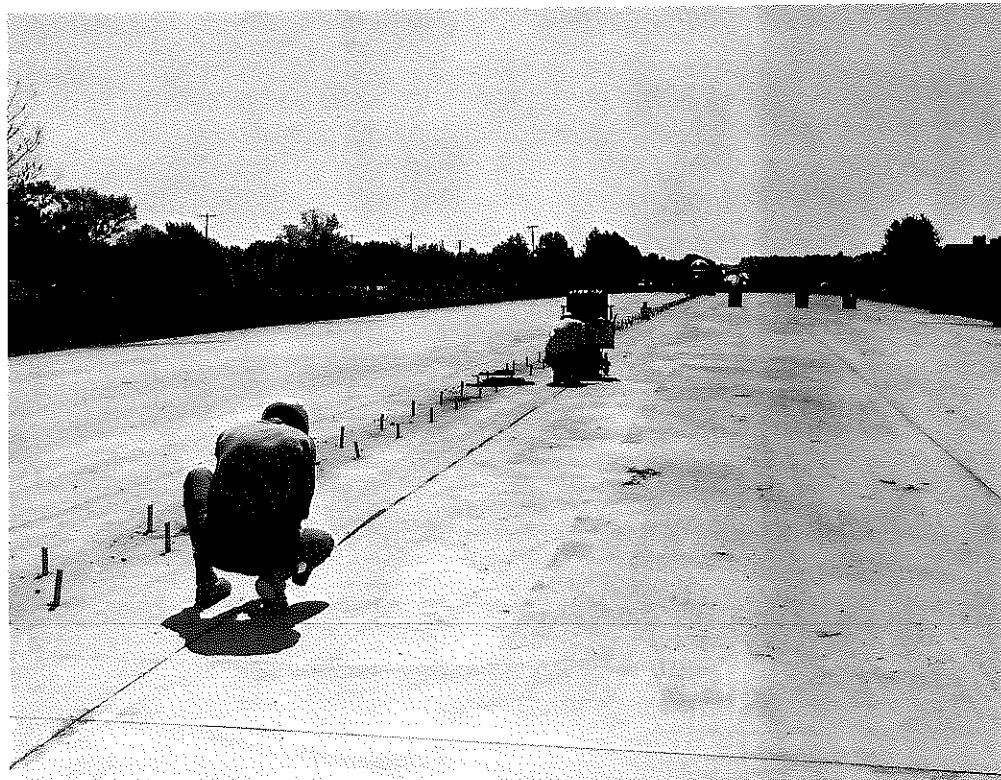
Figure A-18. Installing Neoprene Seal at Inner Edge Joint.
