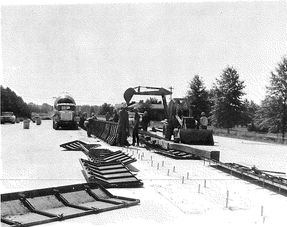
Figure A-20. Installing Median Barrier.
