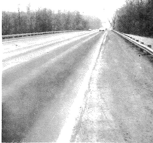
Fig. 9: Porous Sand-Asphalt (Kentucky Rock Asphalt, after Rain; Showing Cleansing of Wheel Paths; Surface Blots readily.
