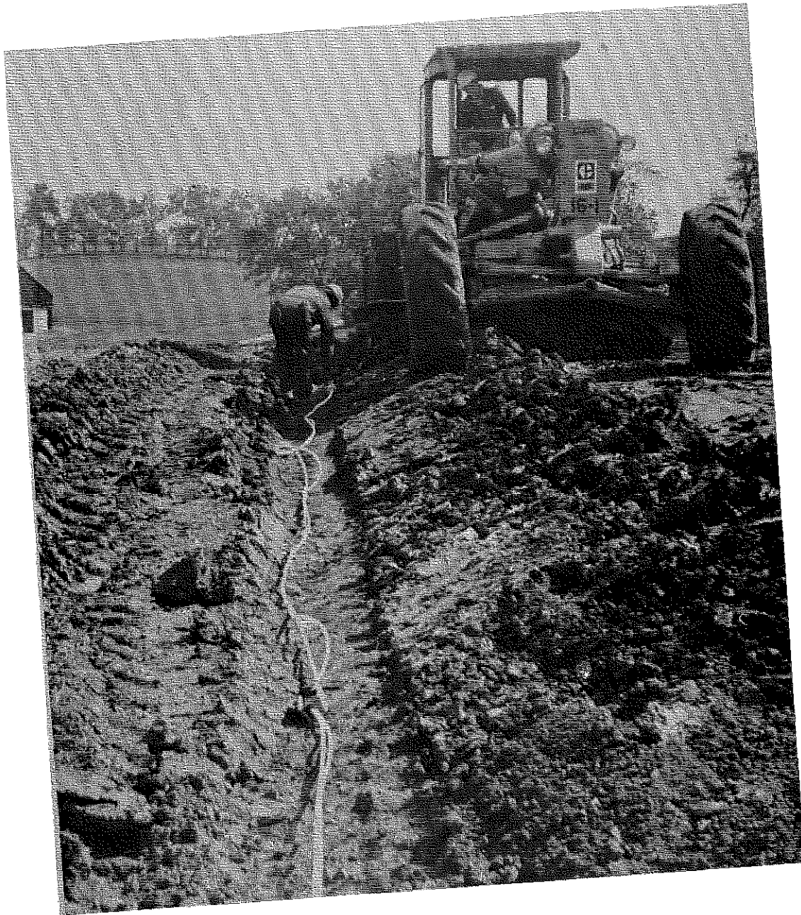
Figure 15. Formation of a Ditch Used in Installing a Settlement Gage.
