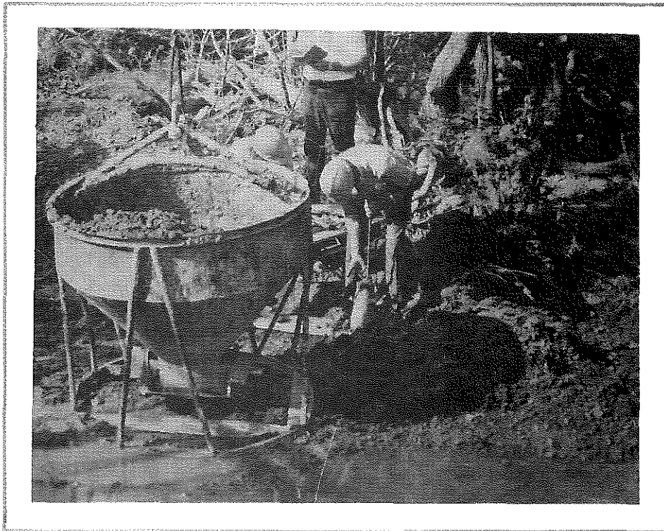
Figure 8. Bucket Used to Unload Concrete, 1/4 Cu. Yd. (0.191 m 3 ).
