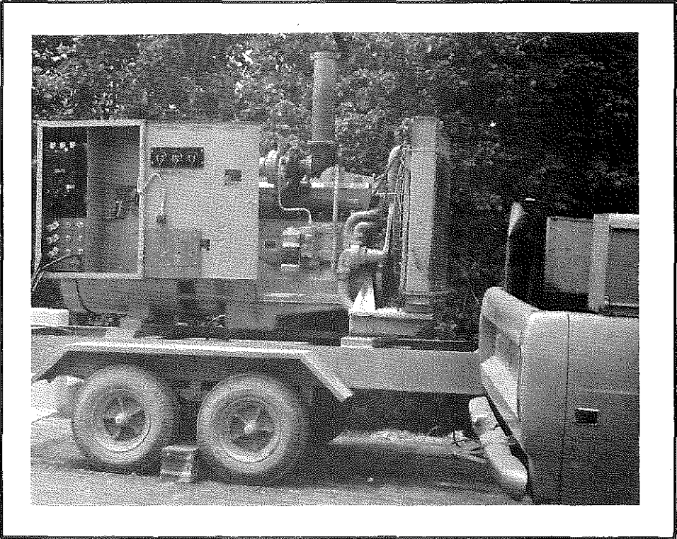
Figure 18. Diesel-Powered Generator Used to Power the Heating Blankets.
