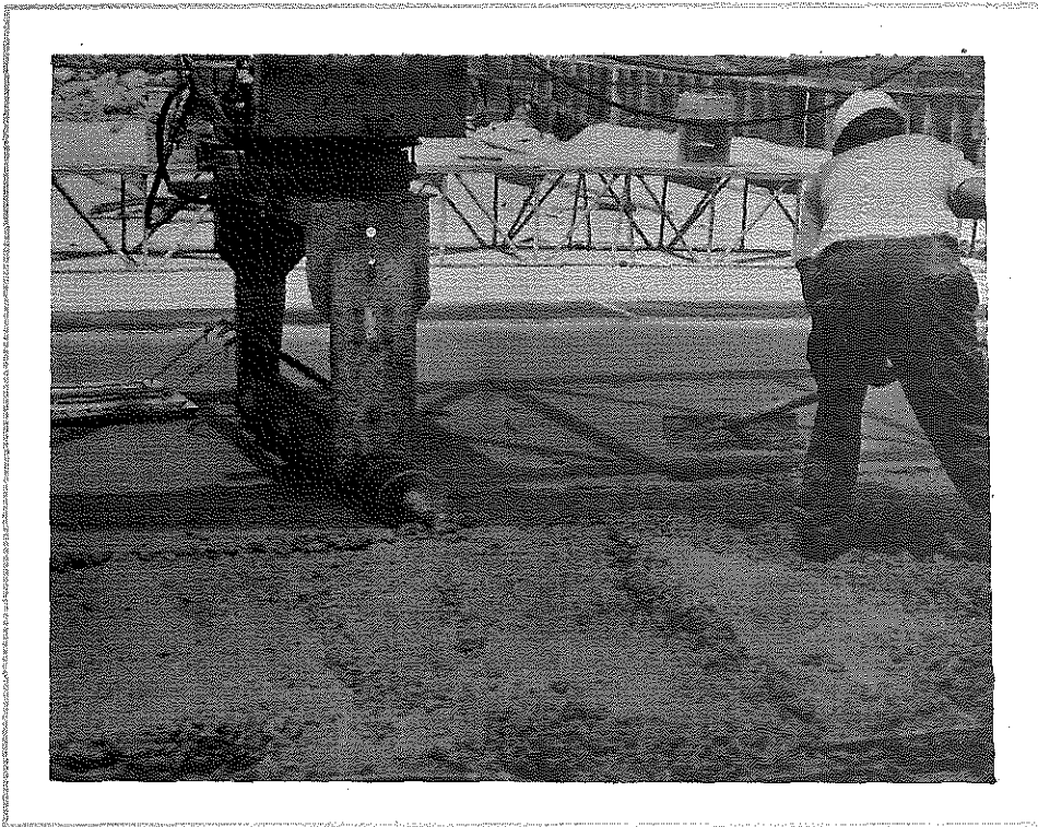
Figure 10. Finishing Drum and Auger of the Gomaco Finisher.
