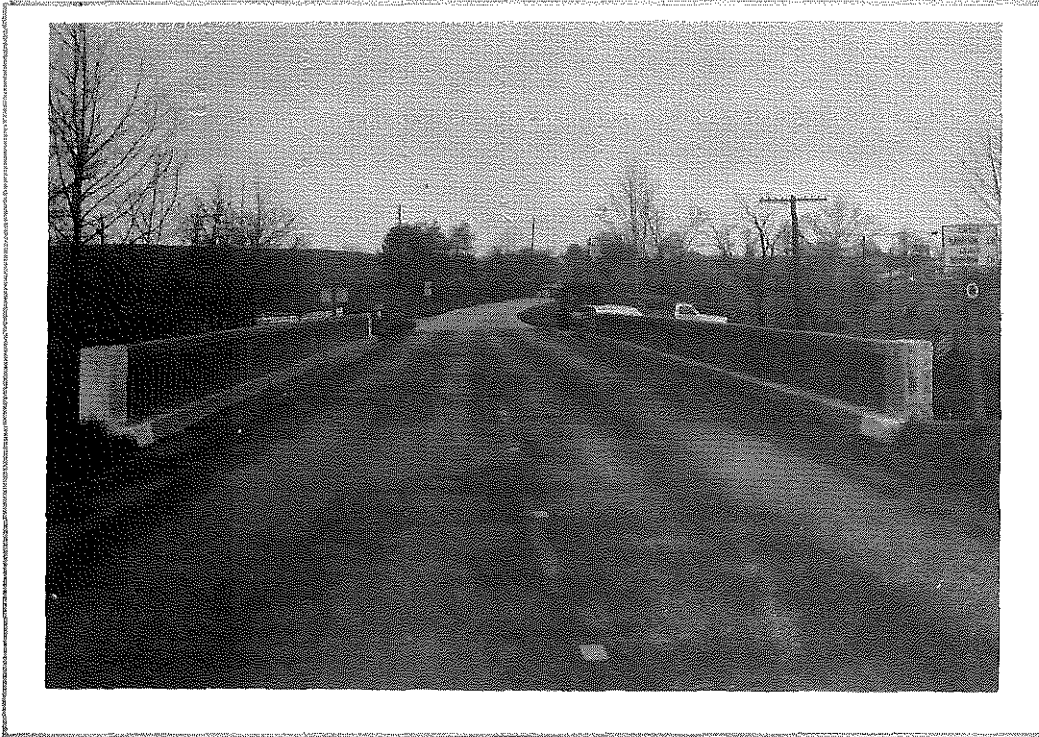
Figure 2. View of the US 27 Bridge over Silas Creek before Reconstruction.
