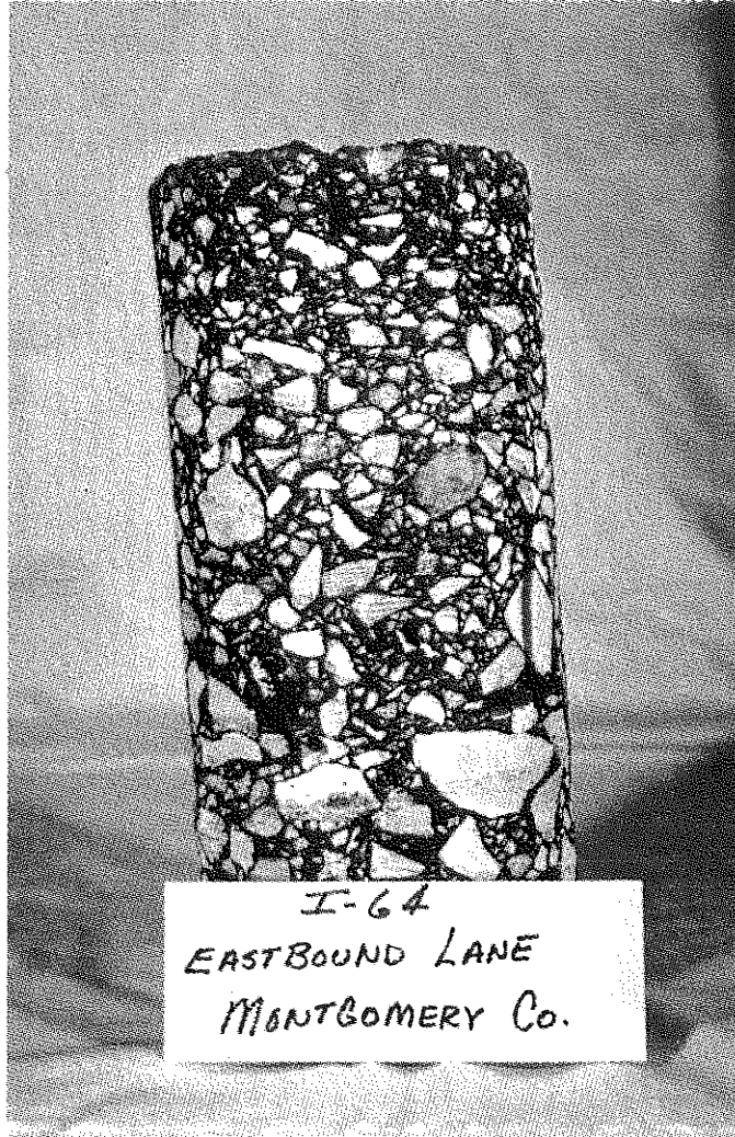
Figure 30. Core Showing Shallow Cracking; Surface Course.
