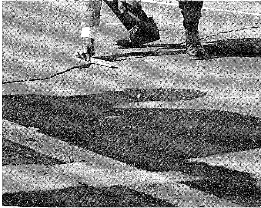
Figure 8. Crack Midway between Contraction Joints which Are Frozen or Locked.
