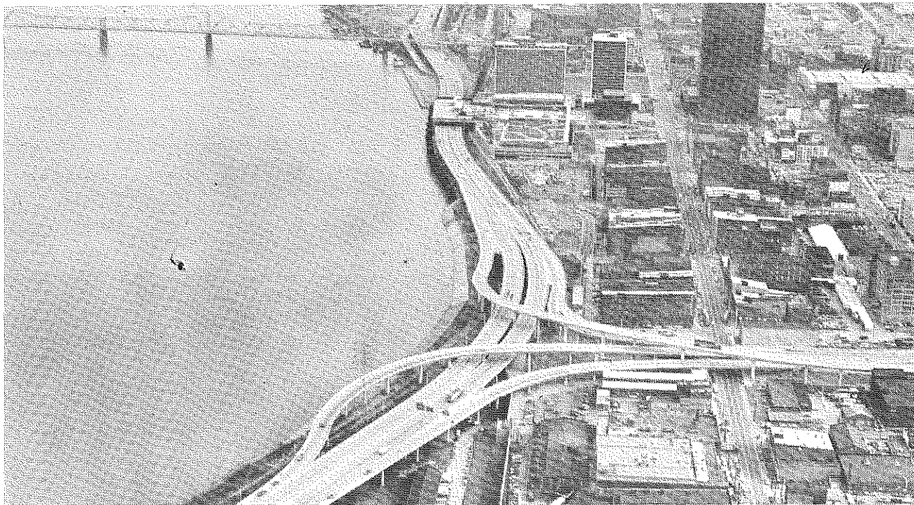
Figure 12. 9th-Street Interchange, Looking Upstream.
