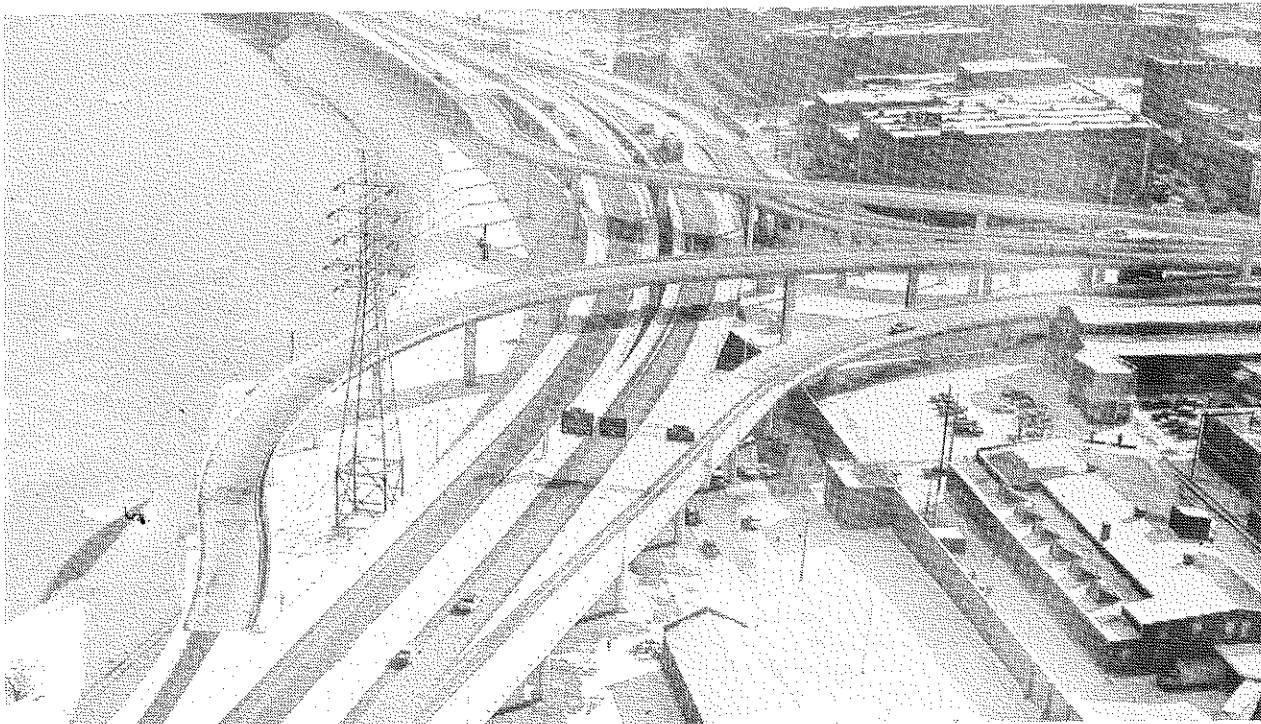
Figure 17. Aerial View of the 9th-Street Interchange on February 2, 1978, Showing the Distinct Difference between Heated and Non-Heated Sections.
