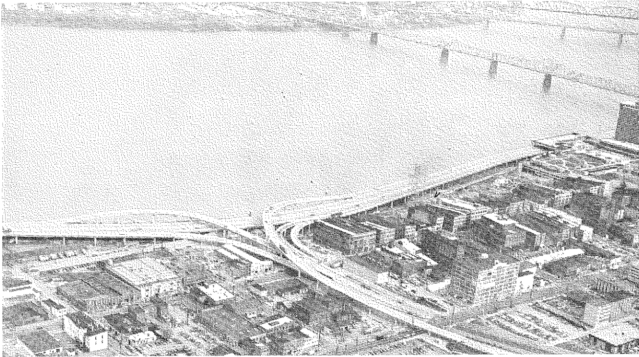
Figure 11. 9th-Street Interchange, Looking toward River.
