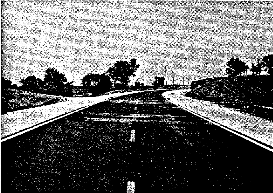
Figure 3. General View of Instrumentation Site at Station 141 + 50 on KY 627, Clark County.
