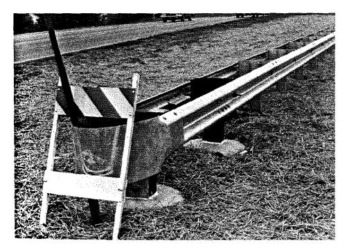
Figure 4. Median-Breakaway-Cable-Terminal (MBCT) End Treatment (Kentucky's Type 6).
