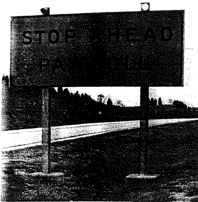
Figure A-11. Rigid sign supports.
