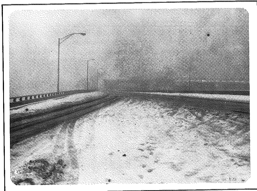
Figure 6. Unheated Pavement (January 14, 1977).
