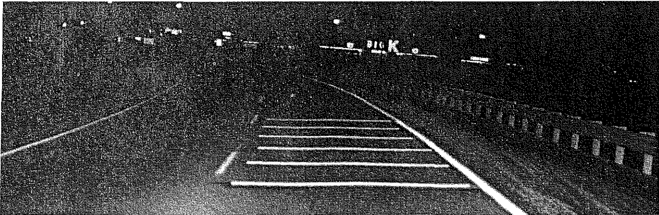
Figure 9. Reflective tape on southbound approach at the intersection of US 127 and US 150 at night.
