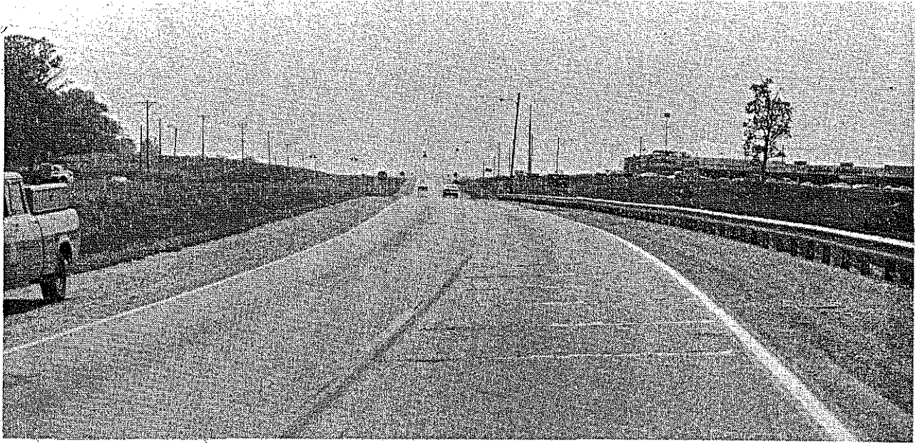
Figure 7. Polyvinyl rumble strips after installation on southbound approach at the intersection of US 127 and US 150.
