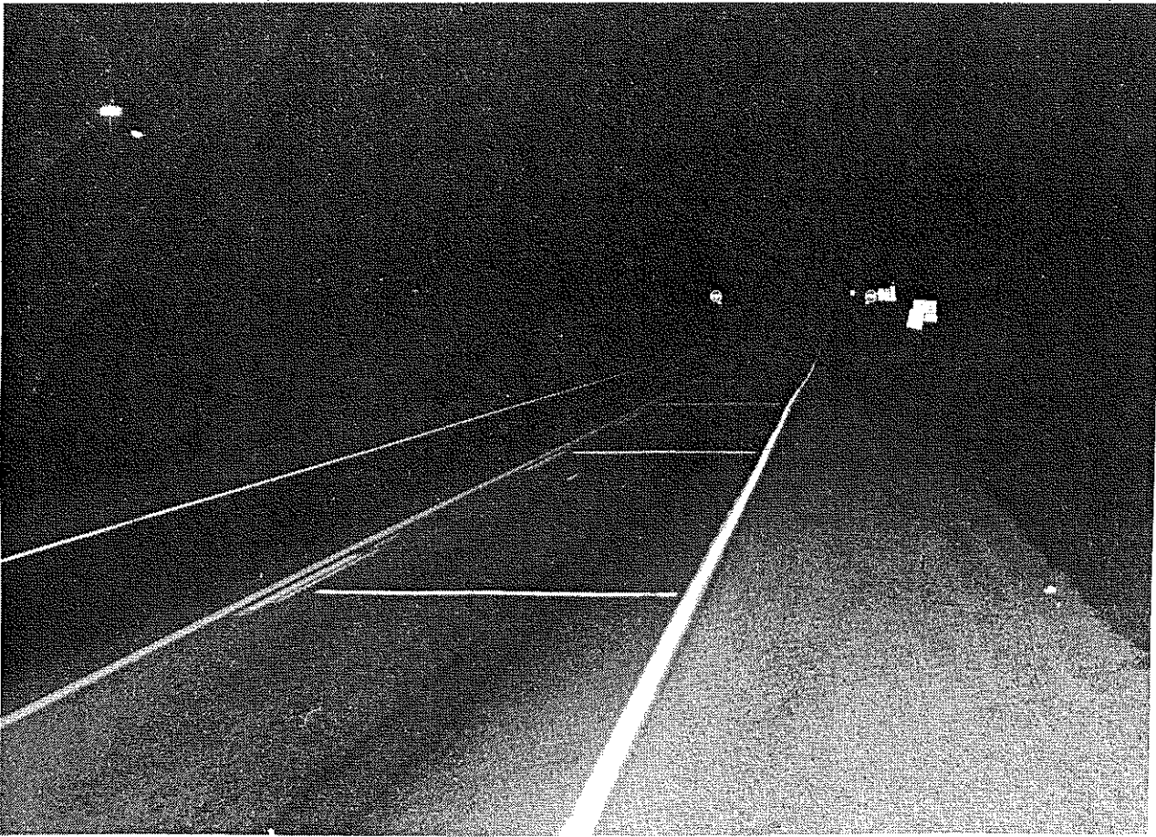
Figure 13. Reflective tape on the northbound approach of US 127 at the intersection of US 150 at night.
