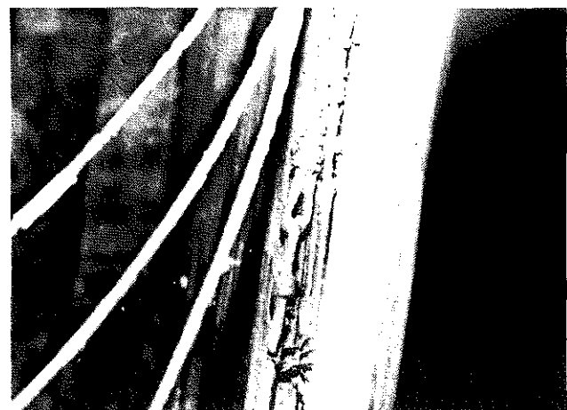
Figure 19. Wire splice in original cable anchor house.
