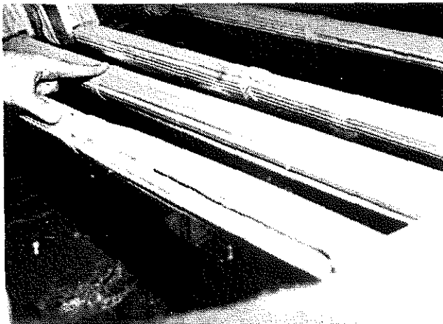
Figure 22. Swollen strands in the downstream Ohio secondary anchor house.
