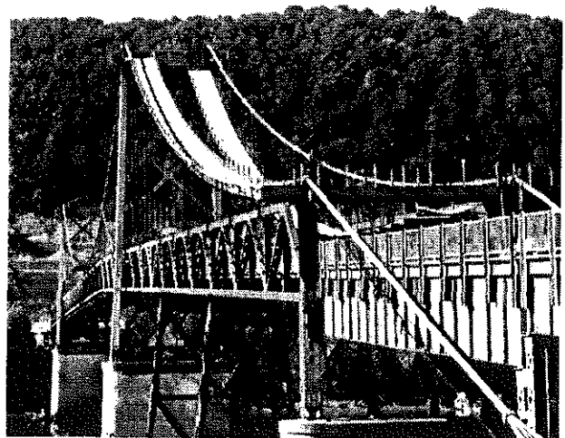
Figure 1. The Portsmouth Bridge early in the recabling operation.
