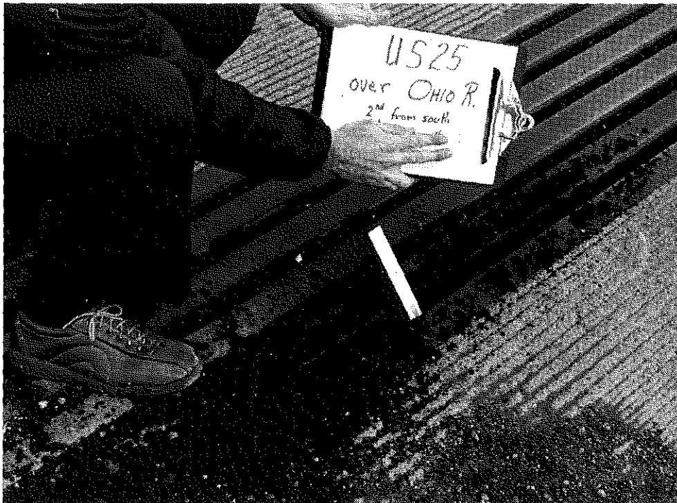
Figure A11. Wabo-Maurer D1300; note debris above seal which is depressed below the pavement surface.
