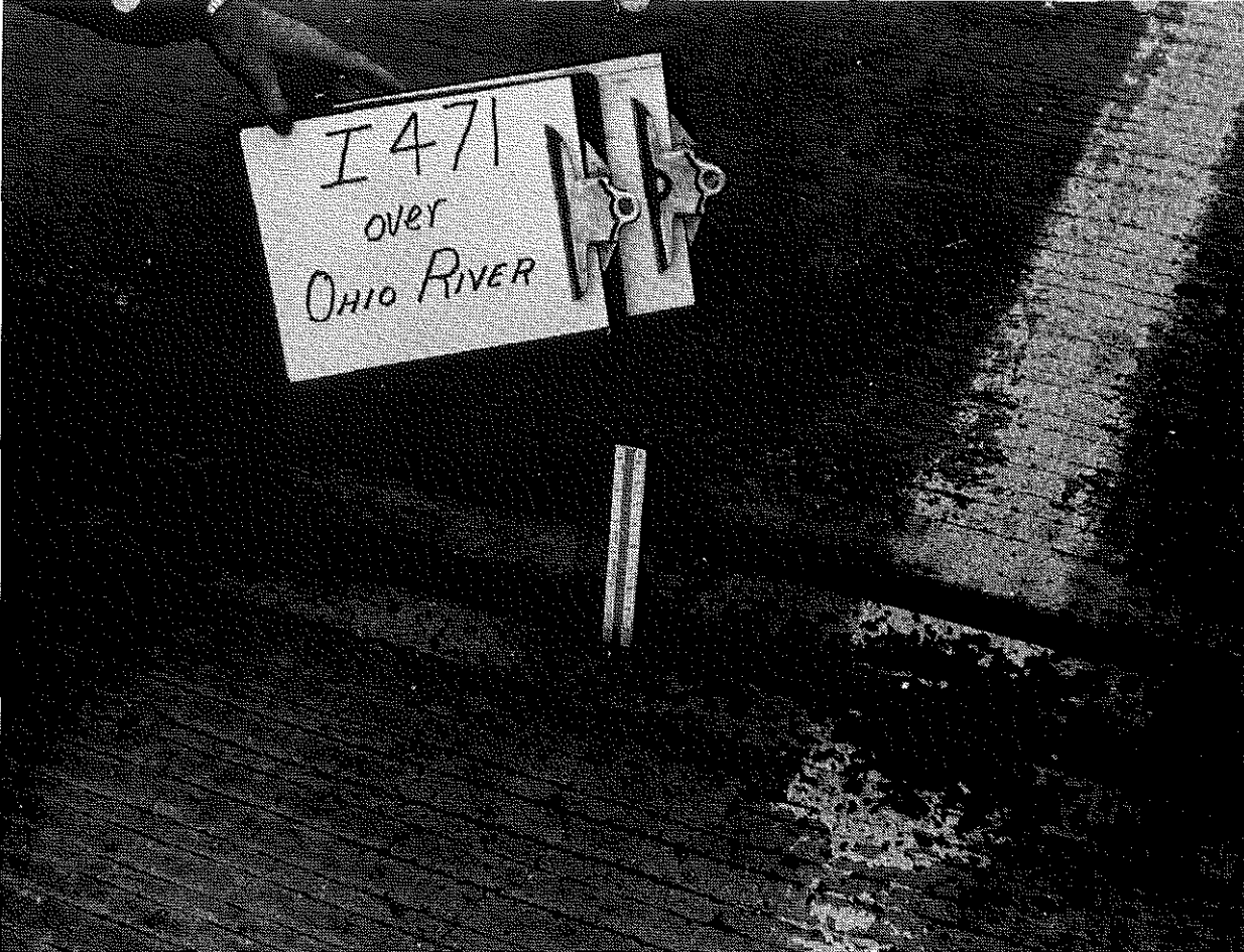
Figure A10. Wabo-Maurer D520; note debris above seal which is depressed below pavement surface.
