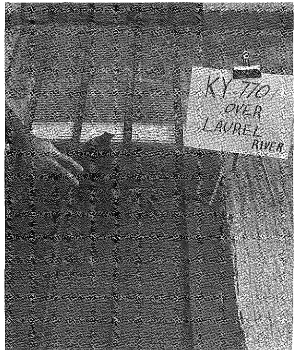
Figure A19. Transflex 650; note tears in the surface of the joint.
