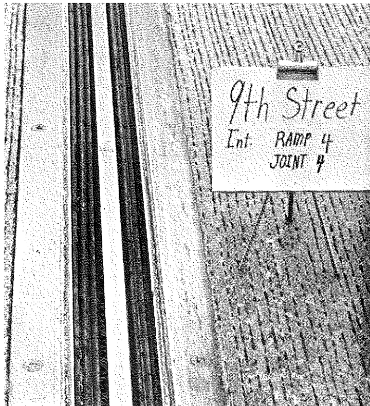
Figure A27. Wabo-Maurer D520; joint in excellent condition.
