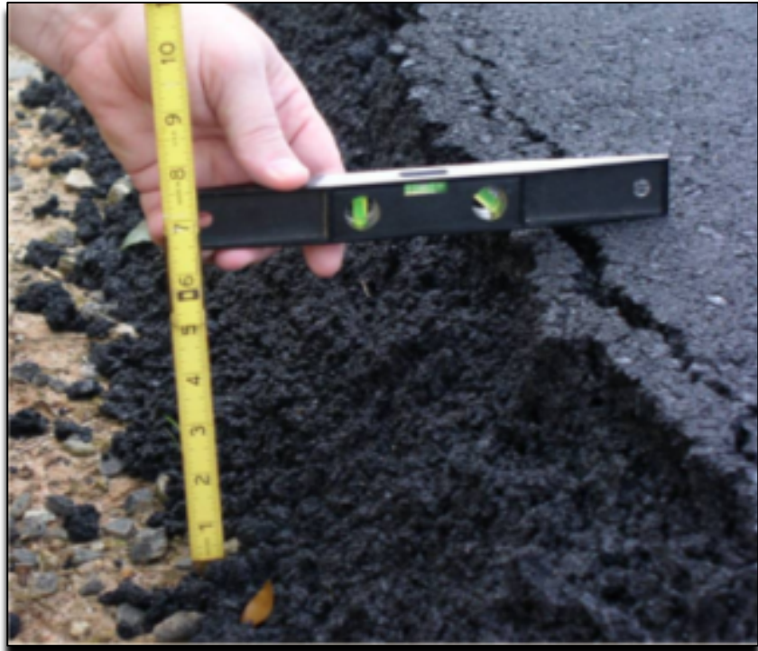
Figure 10: Pavement without Safety Edge
