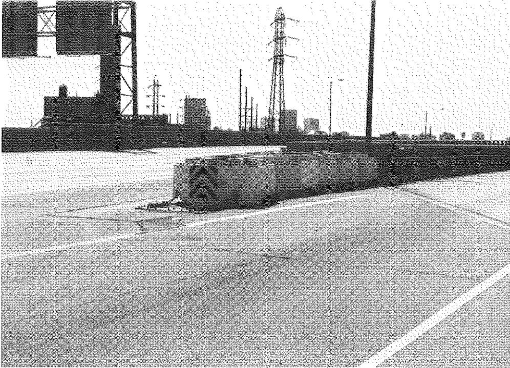
Figure A5. Type V Steel Drums, I 64 Eastbound at 22nd Street Ramp, Jefferson County.
