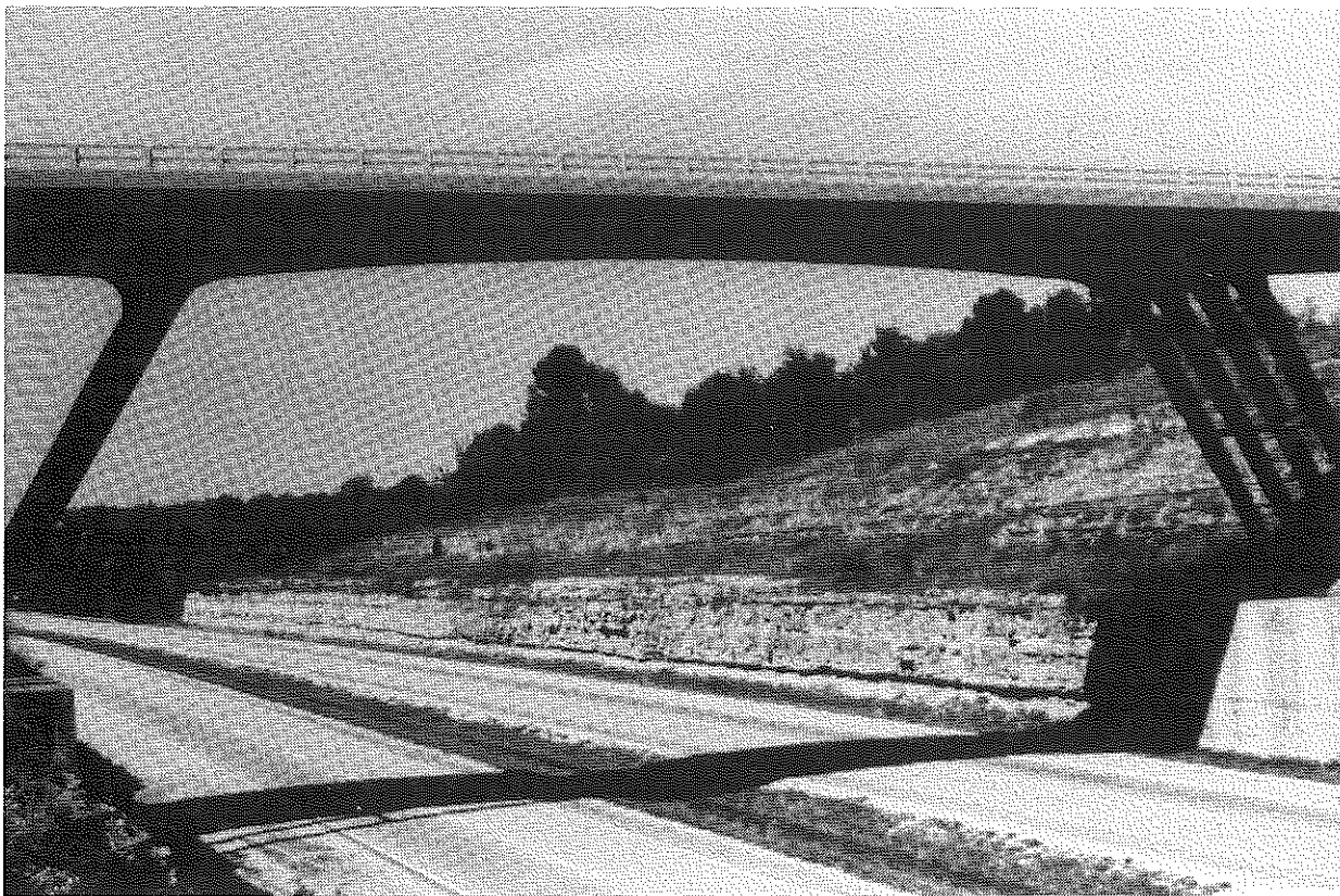
Figure 6. The Scenic Bridge over the Green River Parkway in Warren County.
