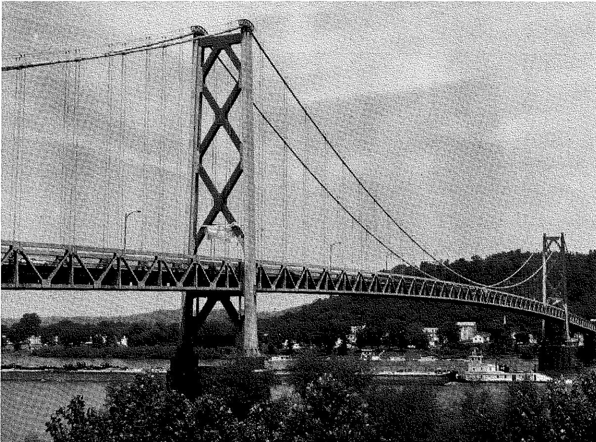
Figure 14. The Maysville Bridge (1977).
