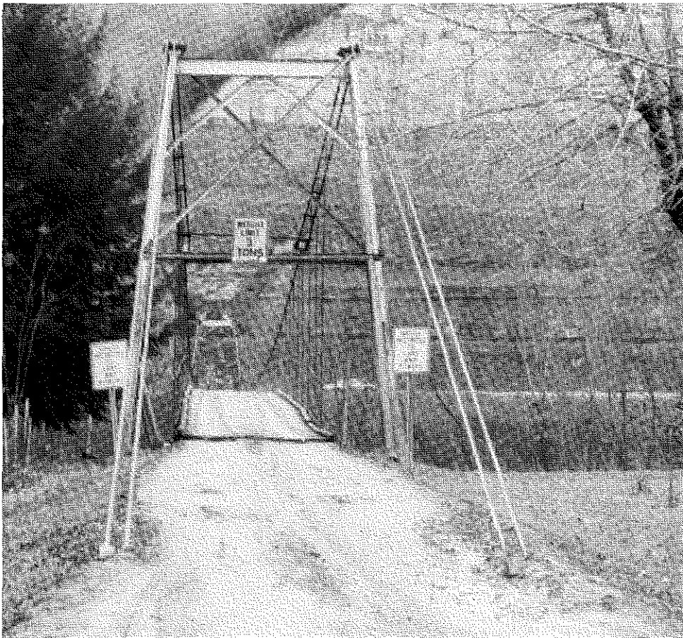
Figure 23. Unstiffened Suspension Bridge in Eastern Kentucky (1982).
