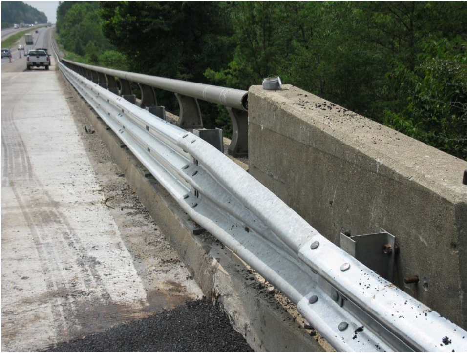
Figure 3.2-Bridge rail retrofit with thrie beam
