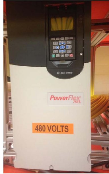
Figure 5.10 Allen Bradley power supply and variable frequency drive.
