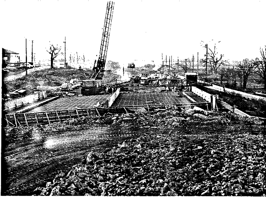
Figure 1: The Construction Site
