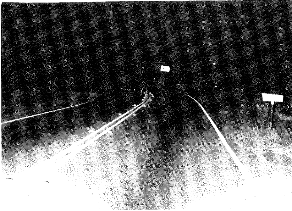
Figure 21. Nighttime Photograph of Blanton Lane After Installation of Raised Pavement Markers.
