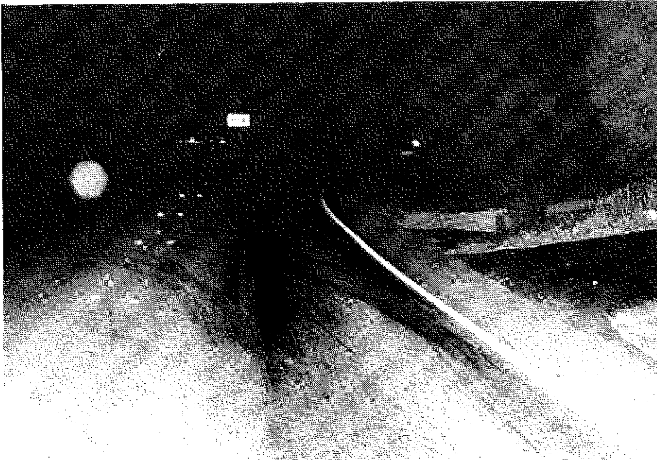
Figure 22. Nighttime Photograph of Fegenbush Lane After Installation of Raised Pavement Markers.
