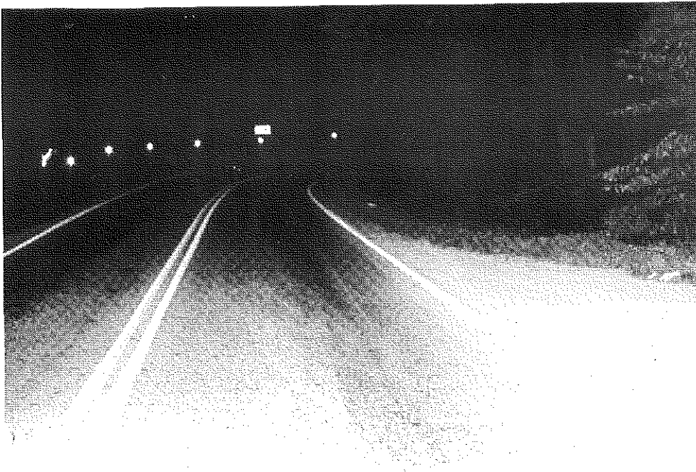
Figure 24. Nighttime Photograph of Post Delineators at US 421 Location Placed in a STD Configuration.
