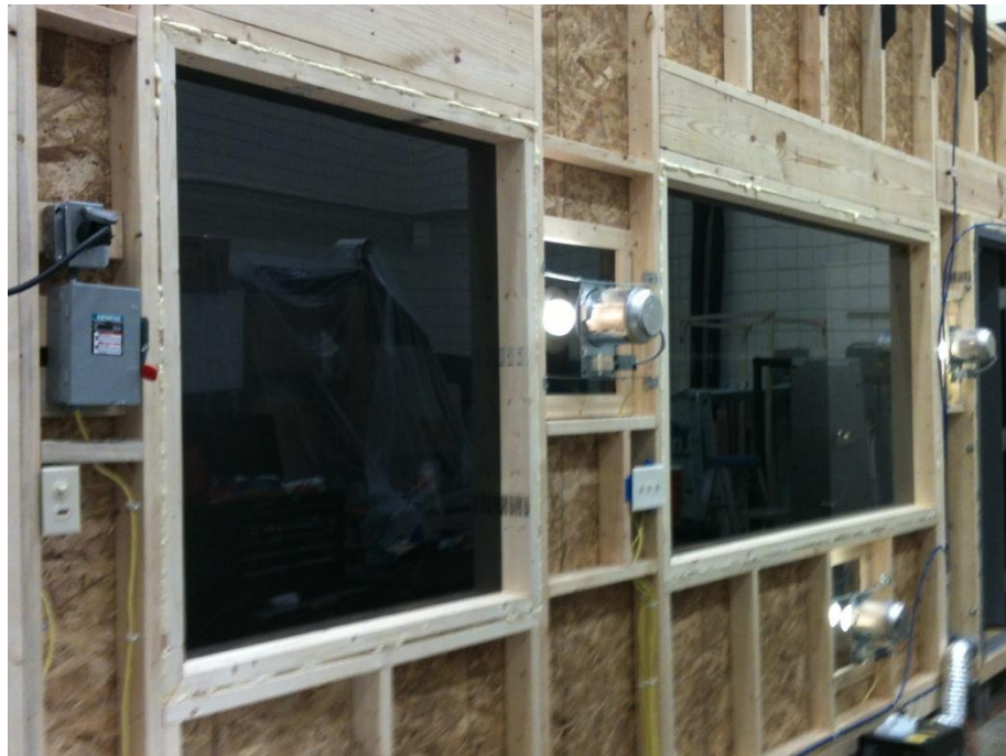
Figure 3-8 – WINTAC: Windows (Inside and outside view)
