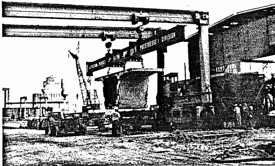
Figure 21. Lifting the Previously Cast Segment from the Car.
