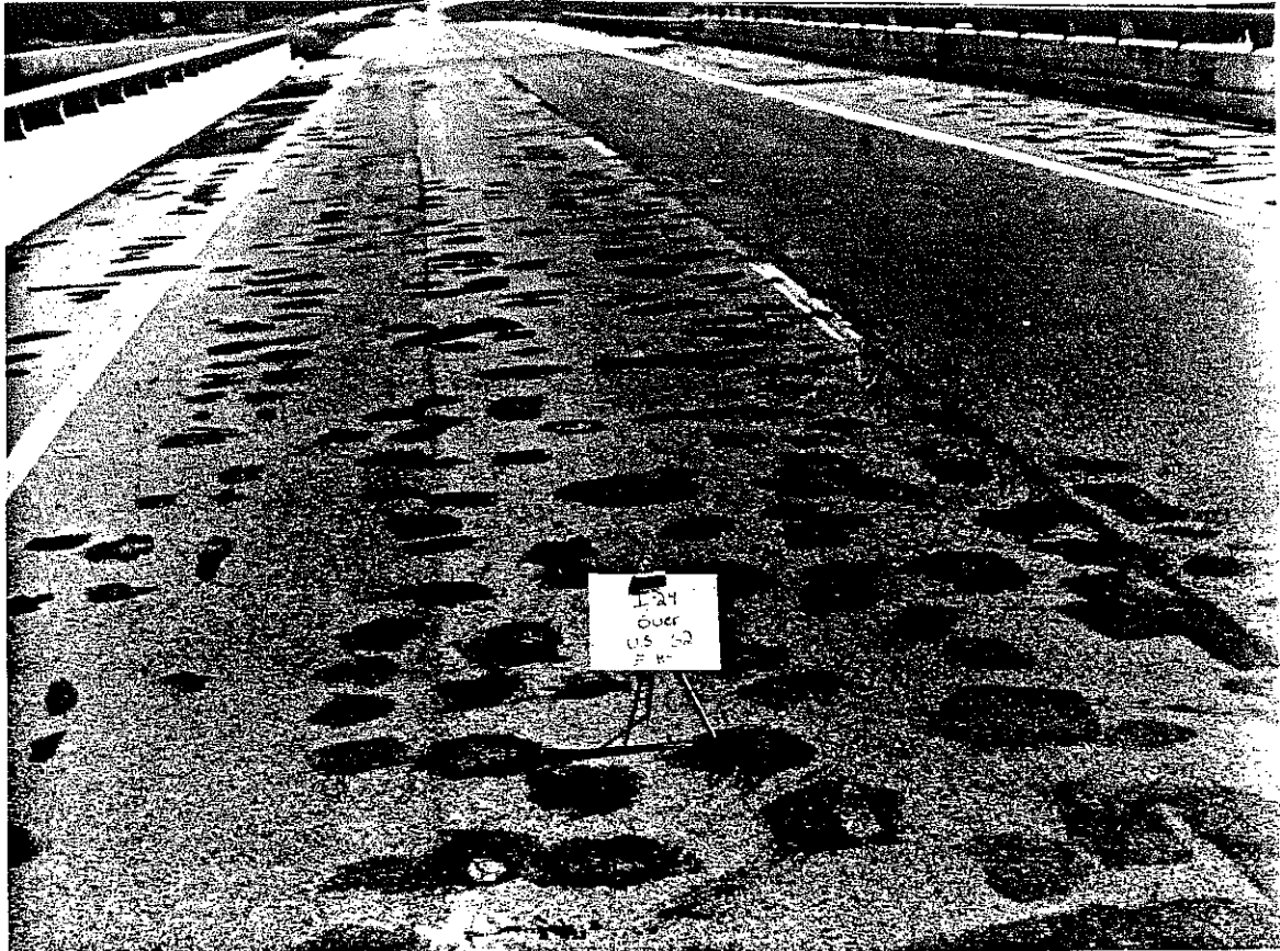
Figure 7. Resealed Blisters on the Membrane of the I-24 Eastbound Bridge over US 62 (1980).
