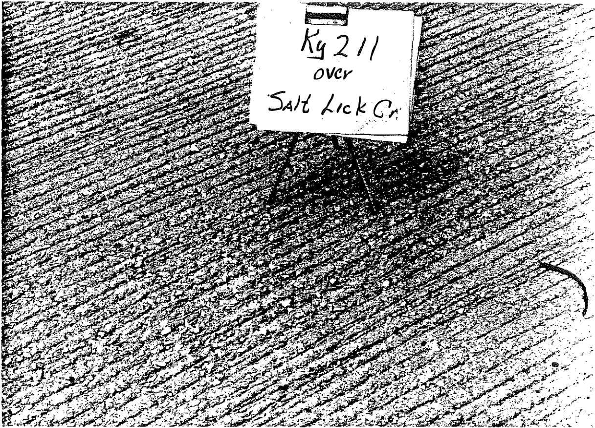
Figure 17. Rough Deck Surface Texturing Caused by Tining (KY 211 over KY 117)(1980).
