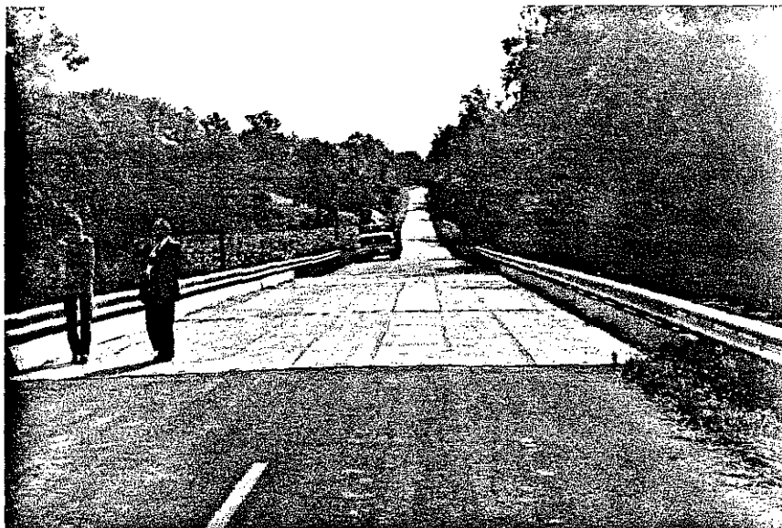
Figure 28. Integral Abutment Bridge Using PCBB Girders (KY 464 over Jonathan Creek)(1984).
