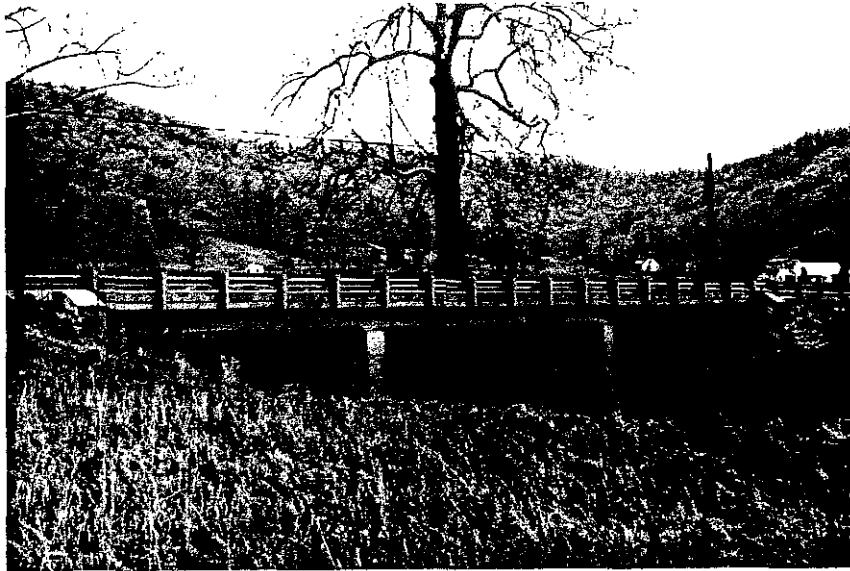
Figure 25. Three-Span RCDG Integral Abutment Bridge (KY 989 over Salt Lick Creek)(1984).
