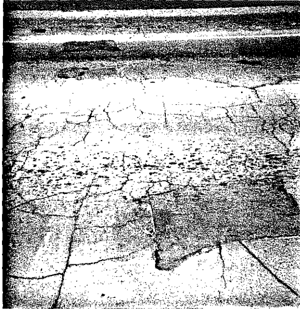
Figure 31. Patch in Concrete Deck Adjacent to Area Showing Block Cracking (US 460 over I 75 in Scott County)(1987).
