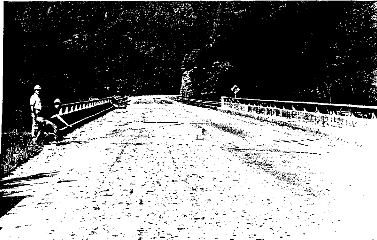
Figure 19. Partially Debonded Dow Latex Overlay (KY 114 over Middle Creek)(1980).
