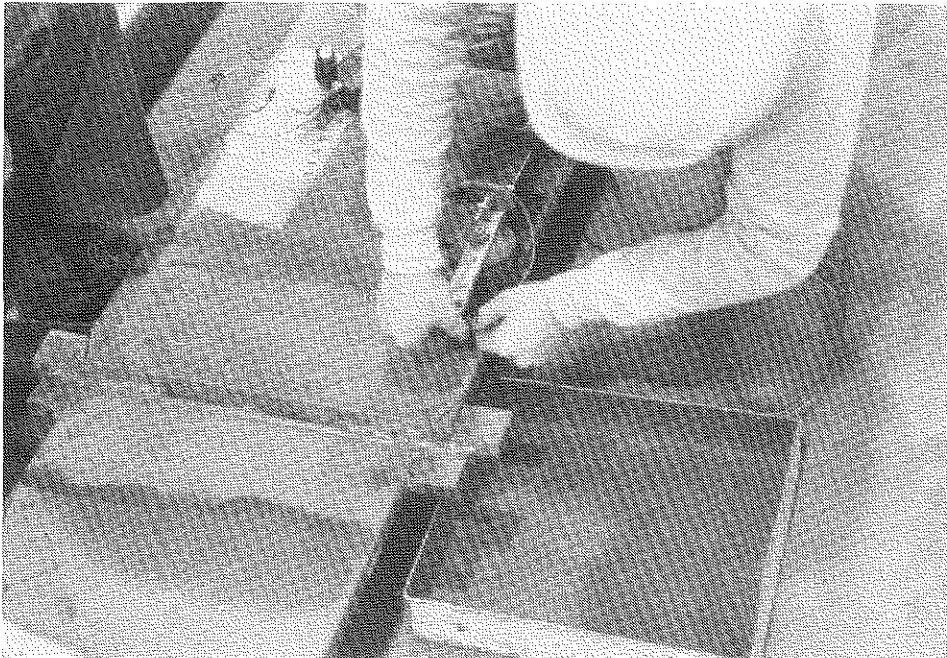
Figure 6. Attaching Transducer to Flange Weld.
