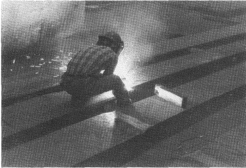
Figure 10. Carbon-Air Arc Backgouging on Back Side of a Flange Weld.
