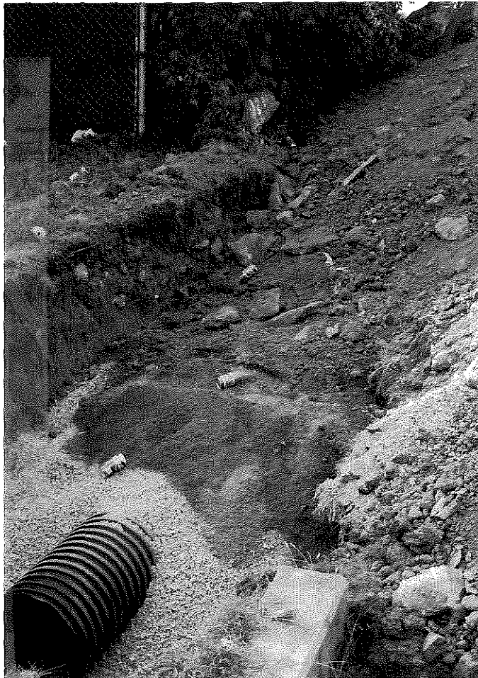
Figure 4. Backfill over Culvert Pipe.
