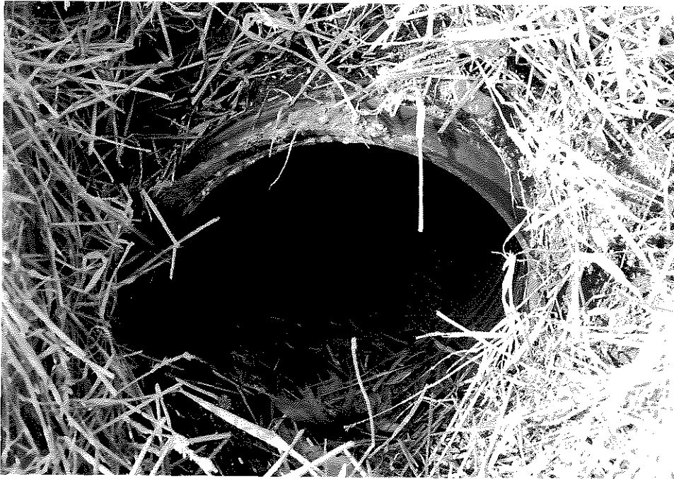
Figure 7. Inlet of Entrance Pipe.
