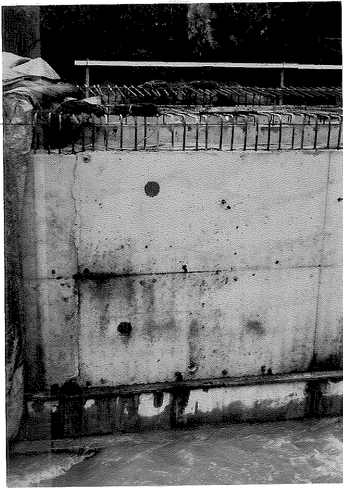
Figure 26. Photo of Sidewall Meters after Forms Have Been Removed.
