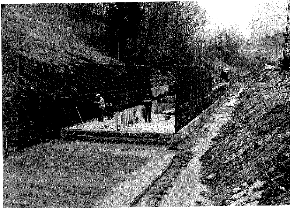
Figure 27. Photo of Culvert 1 (Station 1056+84) Showing Positive Projection, Right Side, and Zero Projection, Left Side.
