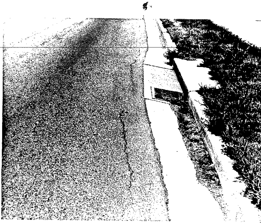
Figure 3. Shrinkage Cracking around Concrete Inlet Drain
