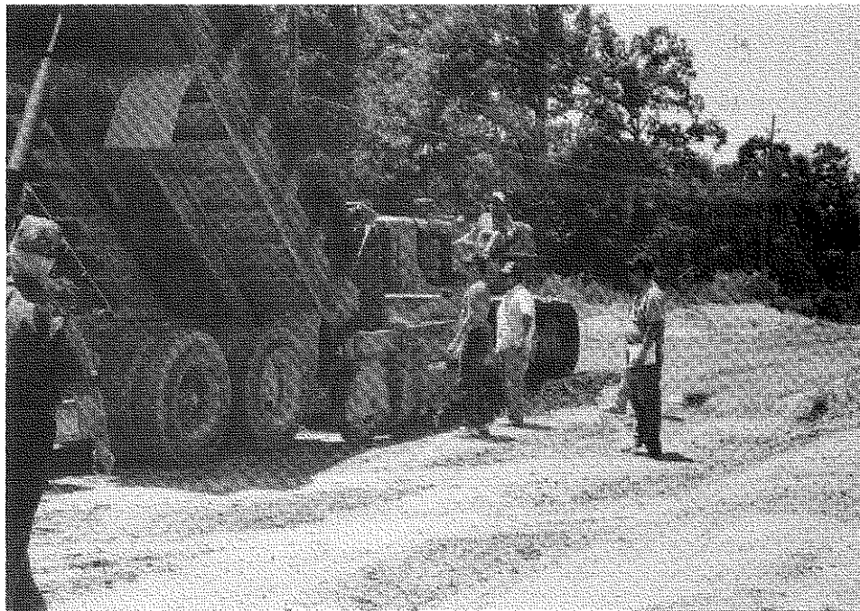
Figure 7. Placing the Experimental Base Material.
