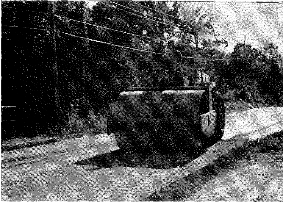
Figure 8. Compacting the Experimental Base Material.
