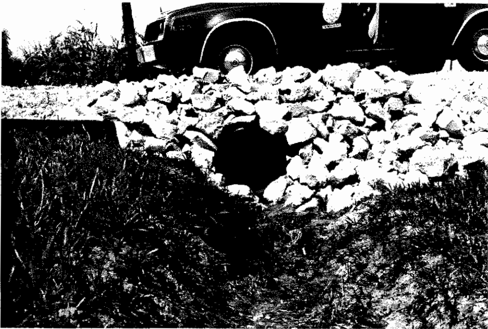
Figure 2. Large Stone Protects Outlet; US 41 A, Henderson County.
