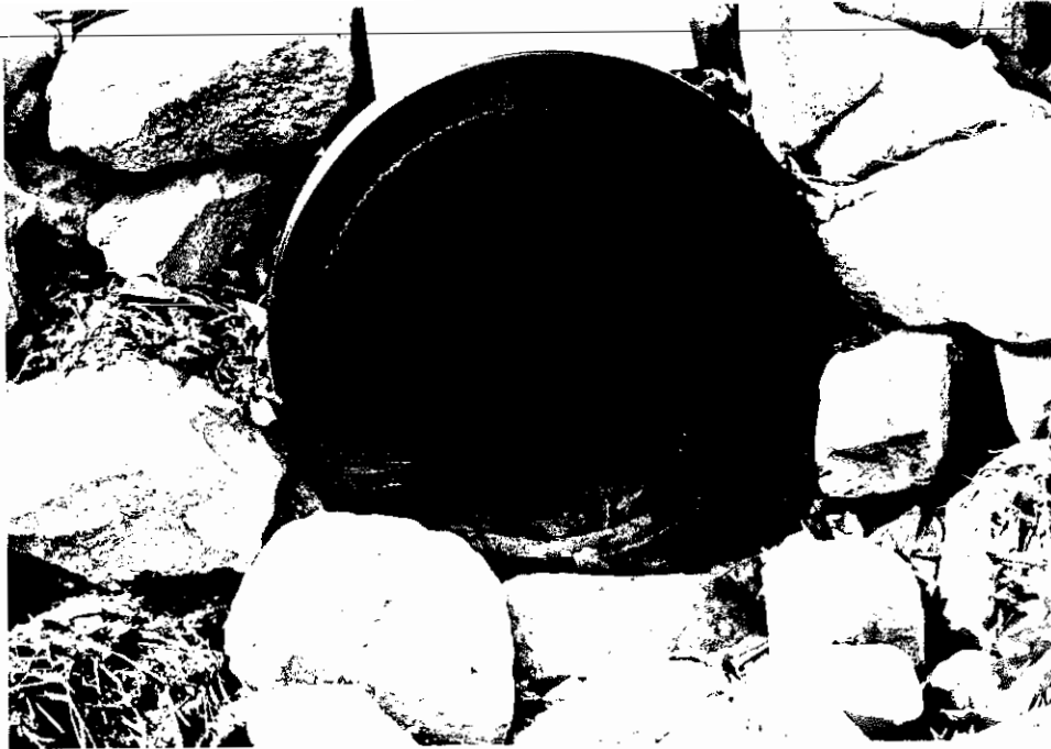
Figure 7. Large Stone Protect Outlet.
