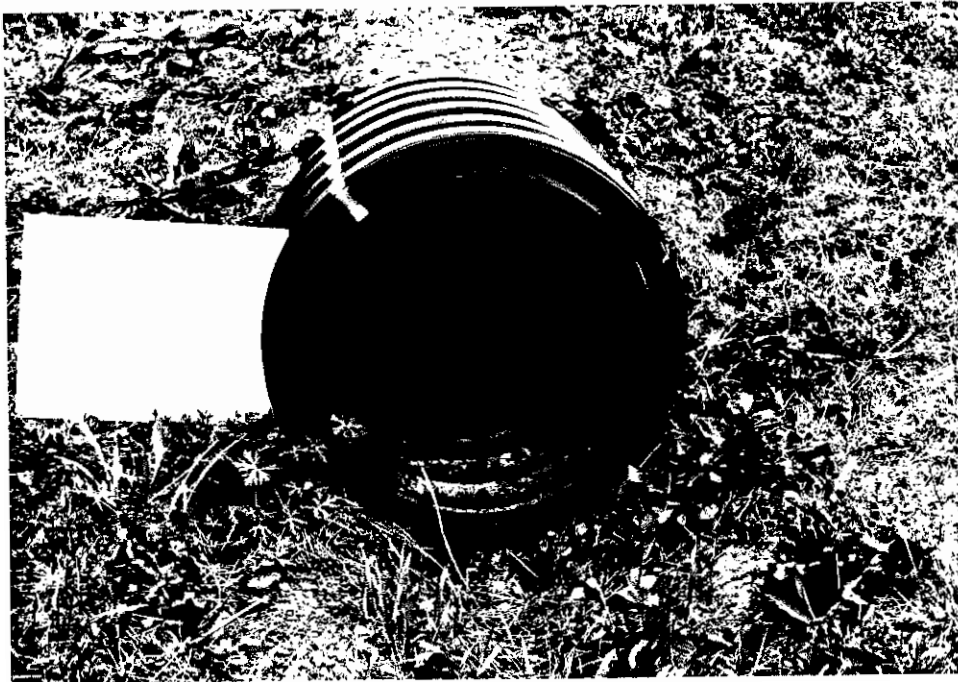
Figure 8. Vegetation Prevents Silting.
