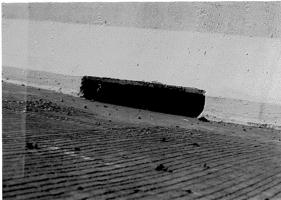
Figure 6. Scupper (Edge Drain) in Good Condition.
