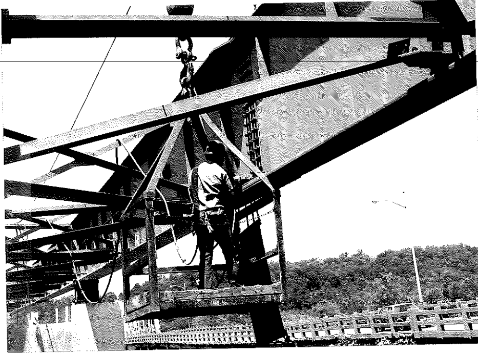
Figure 3. A Workman Installing a LIW/Bolt Assembly with an Air Wrench.
