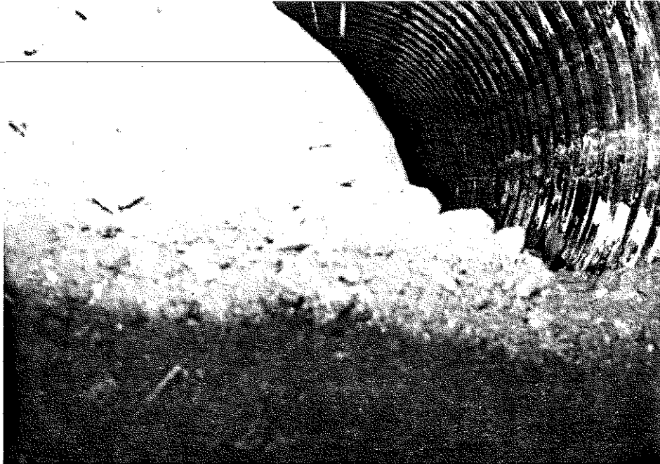
Photo 6. Partially clogged 18-inch pipe.
