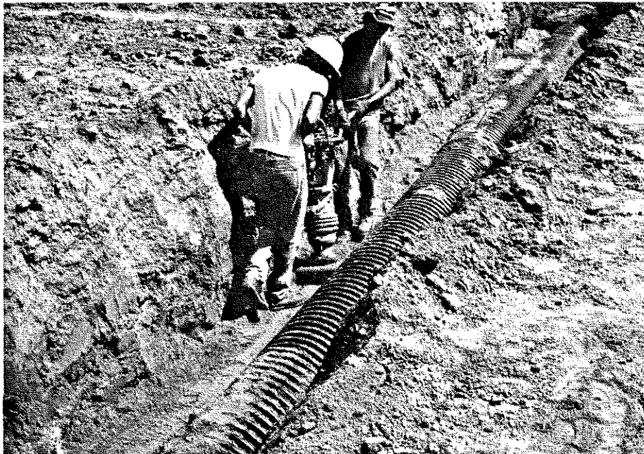
Photo 1. Compacting sand backfill around 18-inch N-12 pipe in Daviess County.
