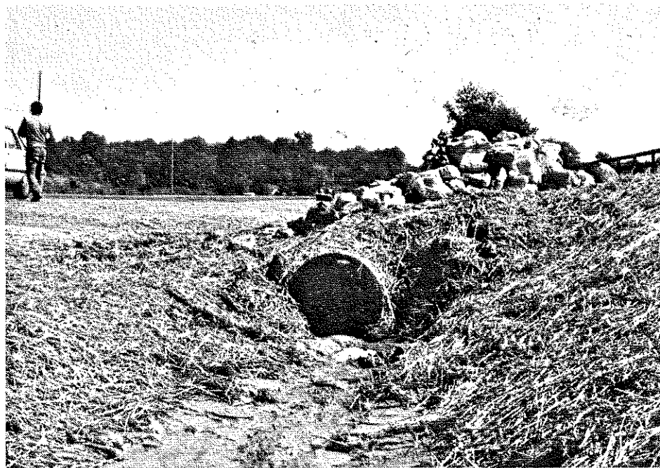
Photo 9. Inloader tracks are present in the thin soil cover above the compressed pipe (Station 167+50).
