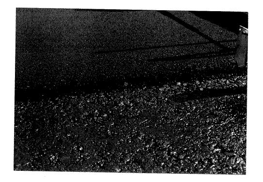
FIGURE 20. TEXTURE OF CLASS K SURFACE WEARING COURSE (BACKGROUND) CONTRASTED AGAINST THE LARGE STONE CLASS K BASE (FORE GROUND)
