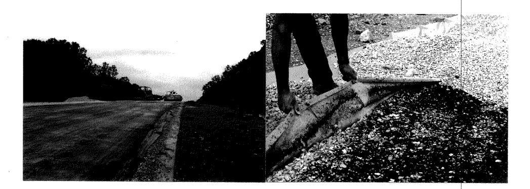
FIGURE 18. SPRAY OF PRIME COAT EMULSION ON THE FILTER FABRIC, A CONSTRUCTION PROBLEM
